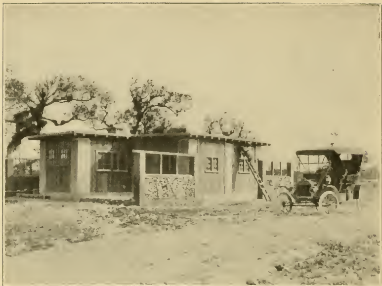
A UNIT HOUSE IN PROCESS OF CONSTRUCTION. CONCRETE ROOF AND CONCRETE FLOORS. THIS HOUSE CONSISTS OF THREE UNITS JOINED TOGETHER ON A TRIANGULAR LOT. VIEW FROM SOUTHWEST.
