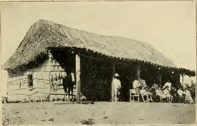
A CUBAN "BOHIO"—A HOUSE BUILT MAINLY OF PALM THATCH.
