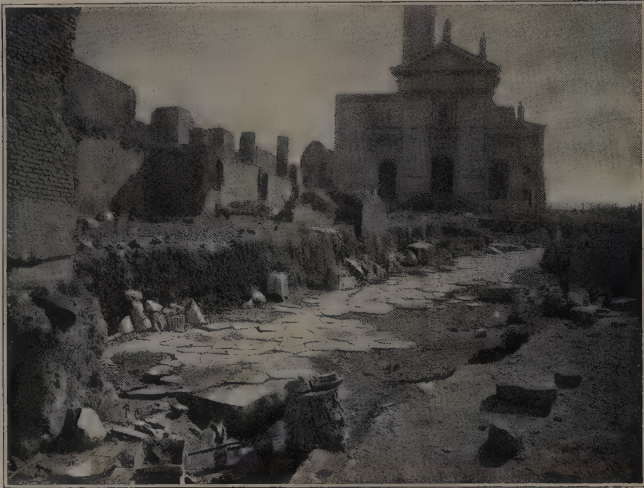
FIG. 64. — THE PAVEMENT OF THE SACRA VIA.
