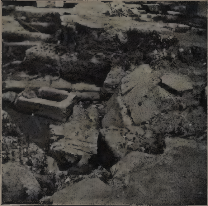
FIG. 52.—SHALLOW PIT, AND VAULT OF THE CLOACA MAXIMA.
