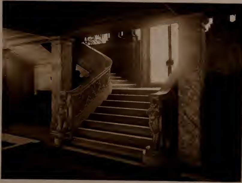
Stairway to Reception Hall
