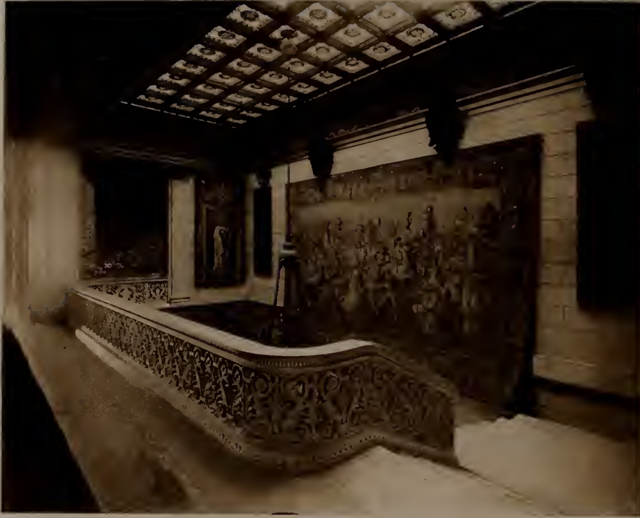
Second Floor Landing
