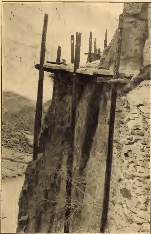
8. Method of constructing a road, or rather, a mountain trail, along the Mekong River south of Yengin. Roads are never repaired until they entirely break down.
