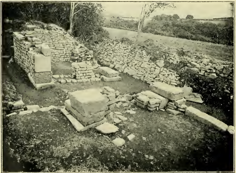
To face p. 29. Fig. 19. South gateway from the north-west after excavation. In right foreground can be seen the sill added when the road-level was raised.
