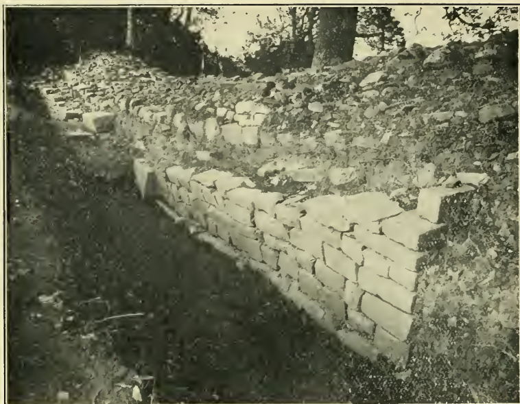
Fig. 24. Back of east gateway underlying post-Roman rampart.
