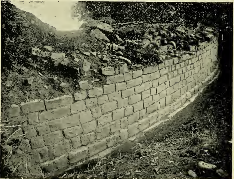
Fig. 7. The fort-wall : south-east corner.
