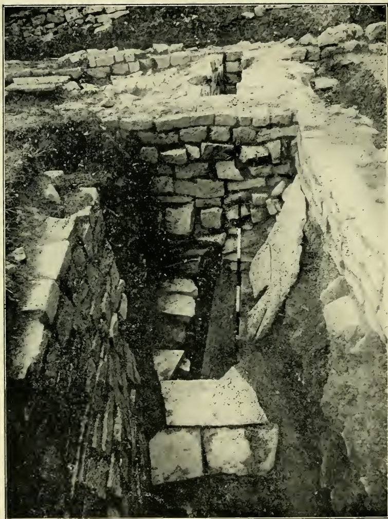
Fig. 45. Building "B": conduit with cover-slabs removed, immediately west of latrine (seen in background).
