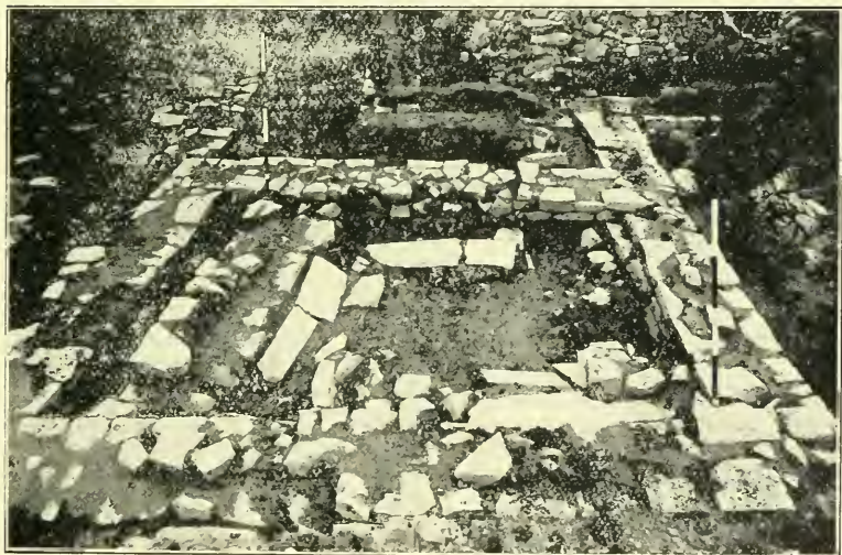
Fig. 44. Building "B": latrine from the east, showing opening into conduit on left.
