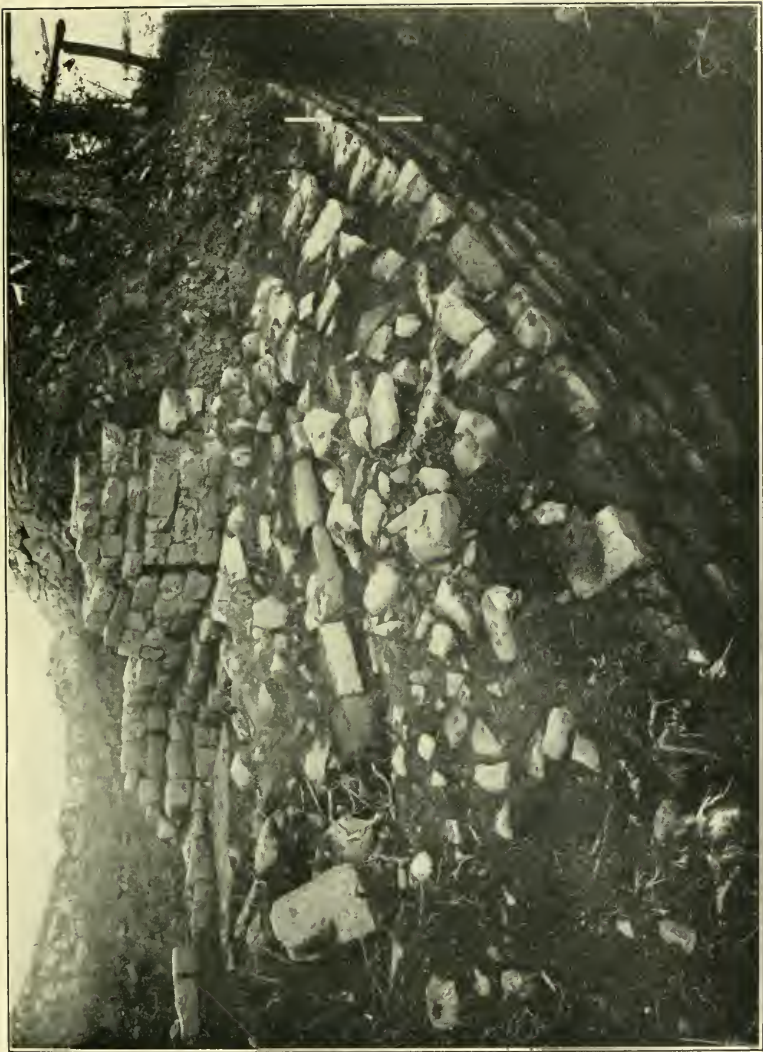
Fig. 27. South-west corner and turret, showing open straight-joint in turret wall.
