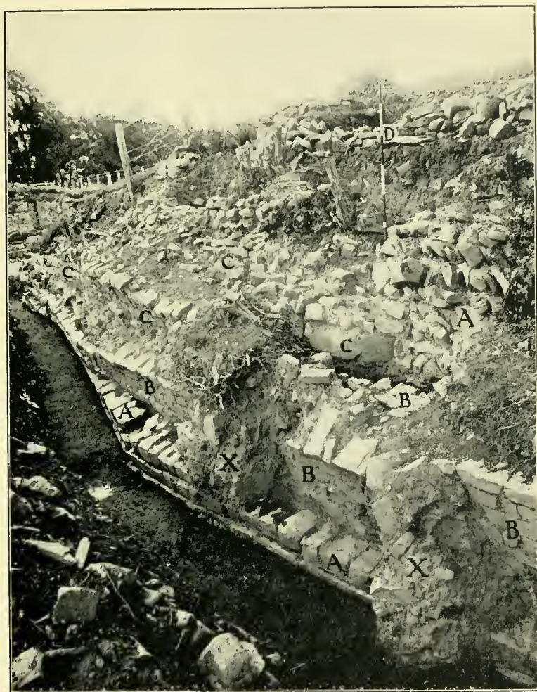
Fig. 9. South wall of fort adjoining south gateway, showing rebuildings necessitated by subsidence.
