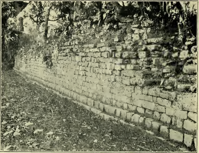
Fig. 6. The fort-wall, north side ; here about 11 ft. high.
