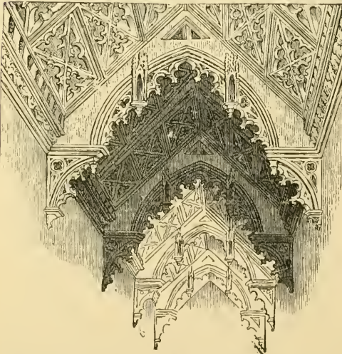
Roof-Supports at Gifford Hall left exposed to the view.
