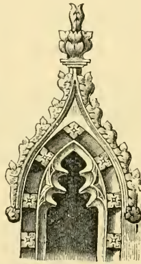
Ogee-shaped Setting of the Pointed Arch, in the Church of St. Andrew at Walpole.
