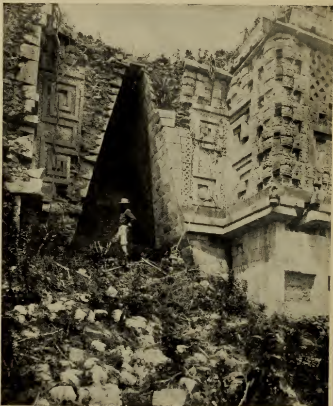
Plate XVII. A Sealed Portal Vault in the House of the Governor at Uxmal, a Building of the Second Empire, probably Thirteenth Century. The vener character of the cut stone comes out clearly. Peabody Museum photograph.
