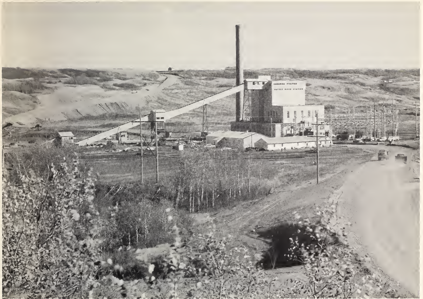
"Battle River Station of Canadian Utilities Limited—First unit 52,000 K.W., coal fired."
