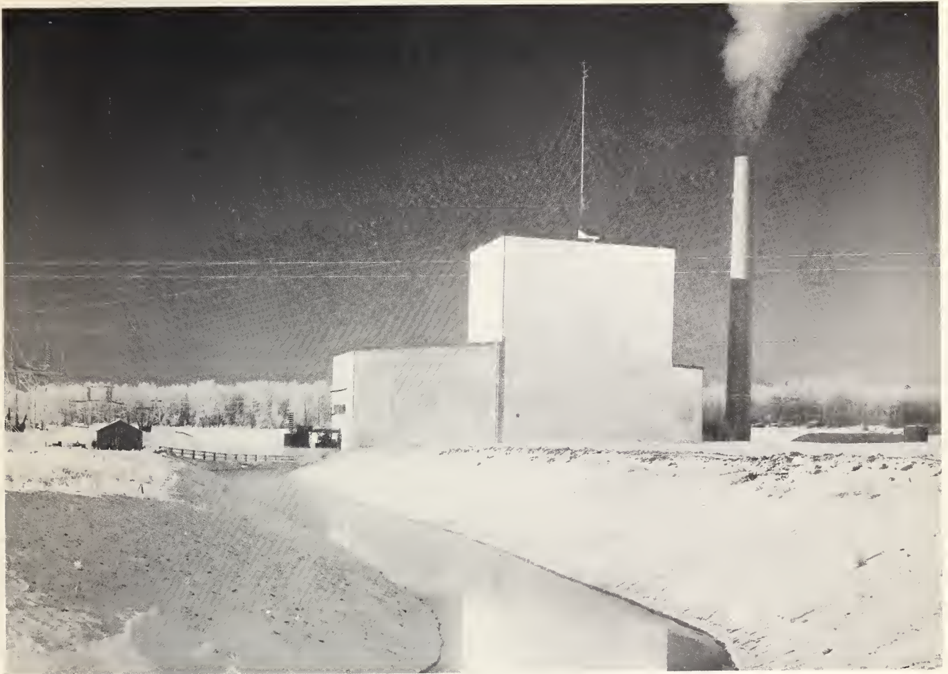
"Wabamun Station of Calgary Power Ltd.—First unit 70,000 K.W., gas fired."
