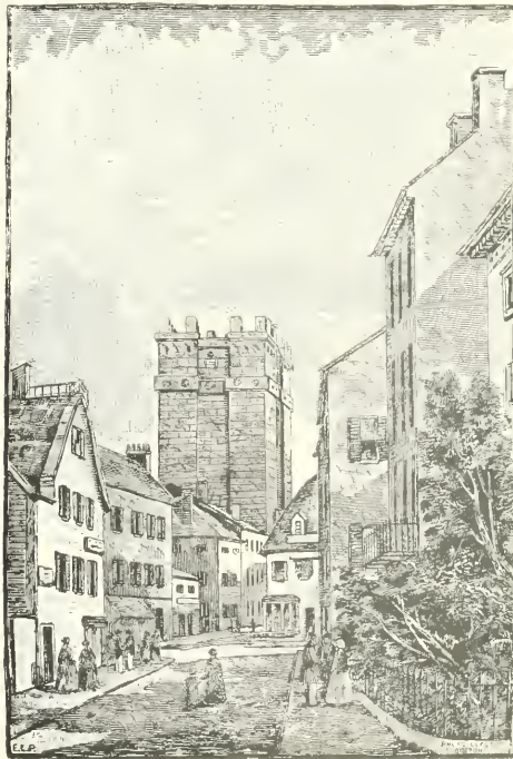
Looking S. E. Junction of Winter, Summer and Washington Streets. Showing second Trinity Church.
