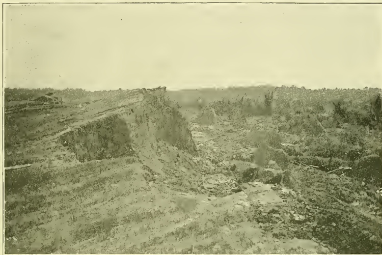
FIGURE 1.—NORTH EDGE OF LANDSLIP AREA, VIEWED EASTWARD FROM NEAR THE OUTLET
