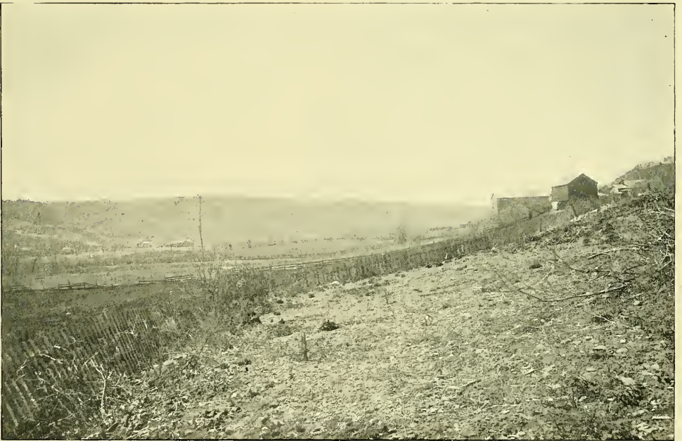
FIGURE 2—VIEW LOOKING NORTHWEST (UPSTREAM) FROM SOUTH ONONDAGA
