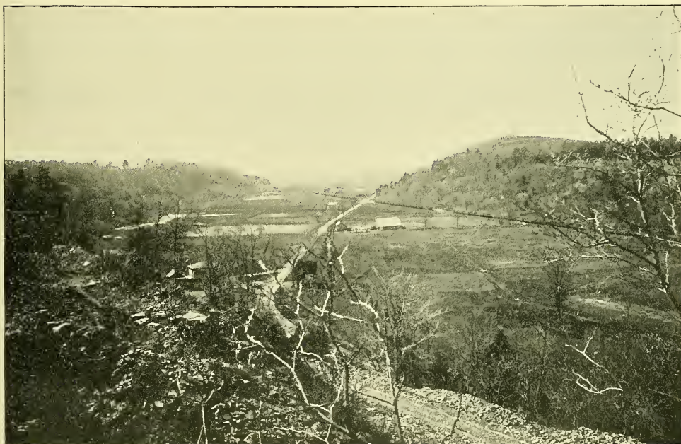
FIGURE 2—VIEW FROM HIGHWAY, SOUTH SIDE OF CHANNEL, LOOKING NORTHEAST (UPSTREAM) Delaware, Lackawanna and Western Railroad in background
