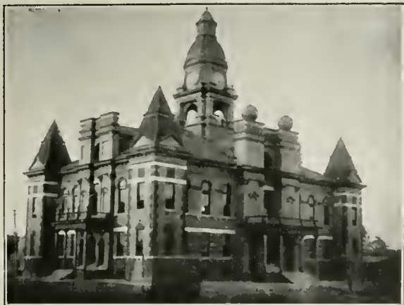
COURTHOUSE AT TRENTON, TENN. Confederate Relic Hall in nearest corner upstairs.
