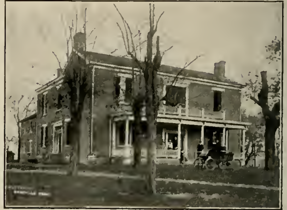
JOHNSON HOUSE. East of pike midway between Franklin and Brentwood.
