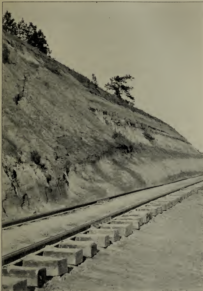
CUT SOUTH OF STATION, COLUMBIA, LA.
