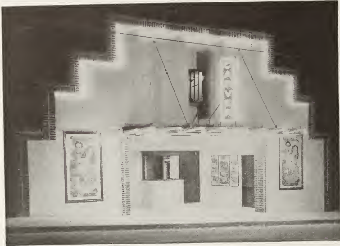
The Quonset construction extends to the brick and stucco front.
