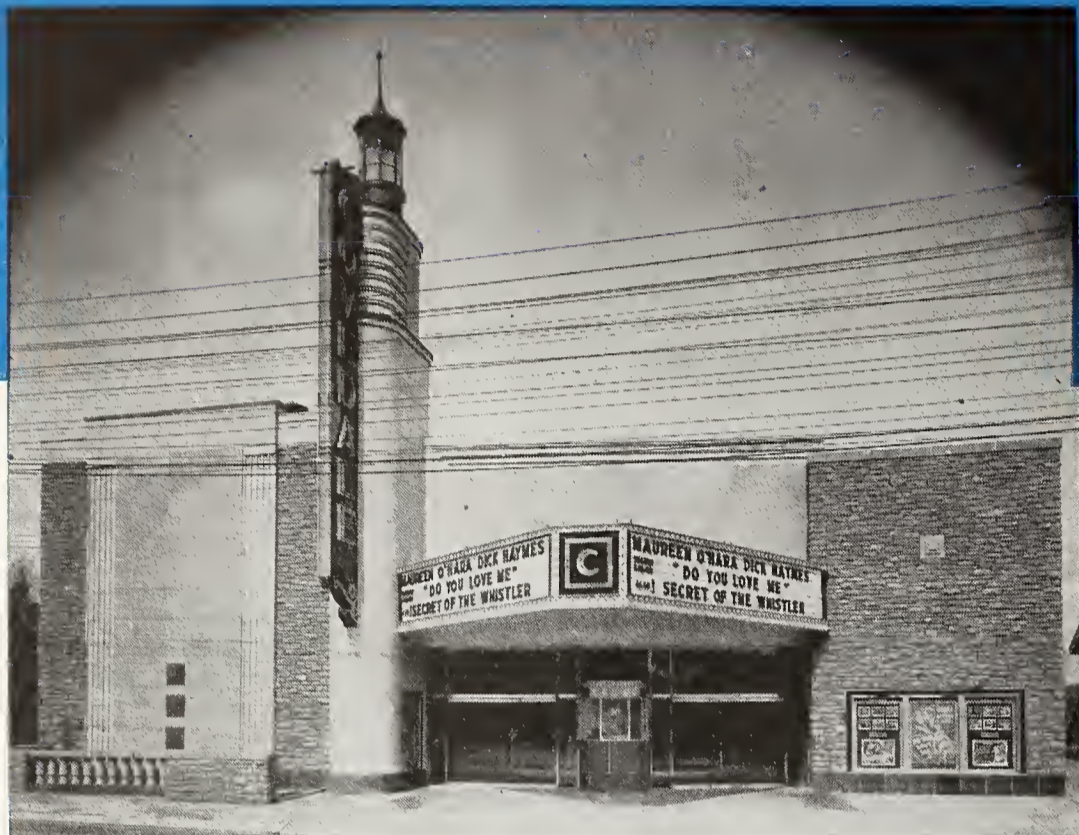
■ The Covedale theatre, which becomes the third house owned and operated in Cincinnati by Ackerman Enterprises, has a front combining terra cotta and native rubble stone in an architectural effect advised by the fine residential section it serves.
