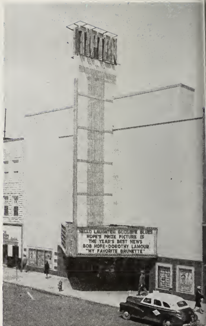
■ Of radically different location from the Covedale is the Tipton theatre, which has been designed to be conspicuous among the institutions of Huntington's central business section. Executed mainly in terra cotta, its front is severely modern in a simple massing of two walls tied together by a tall sign fin. The Tipton is owned and operated by Abe and Sol Hyman.
