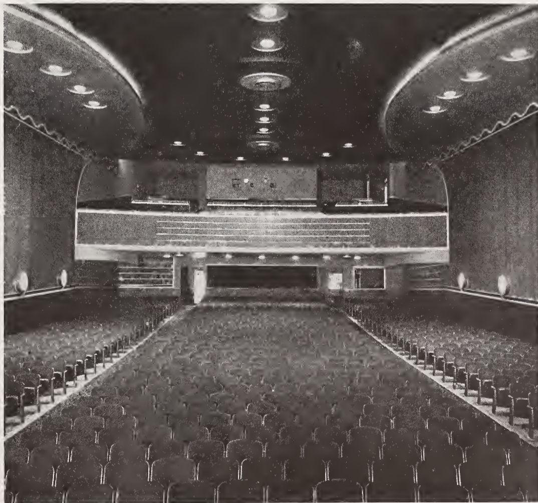
The auditorium of the Tipton theatre has sidewalls of fibreglas fabric, in wine color above a plum-colored wainscot. Pattern is supplied largely by the ceiling, with its numerous circular light troughs, some of them suspending Agitair air diffusers.
