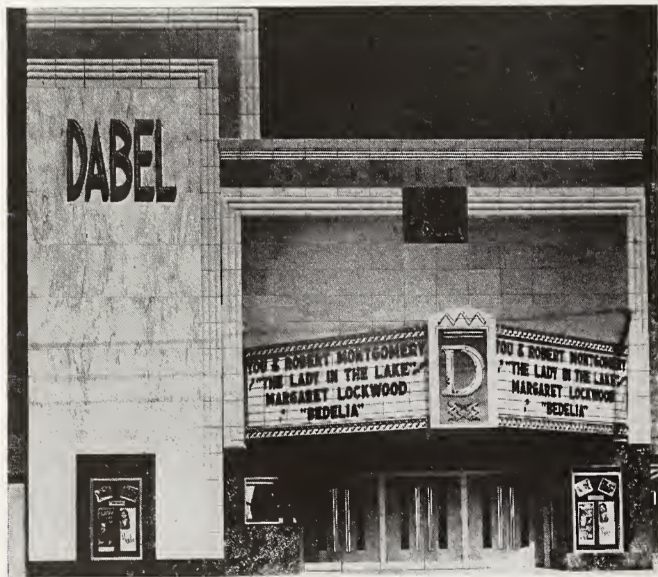
■ The Dabel, like the Covedale, is a neighborhood house, but its location is in a community of industrial workers, to whom it has been designed to bring motion picture entertainment in an inspiring environment. Its front combines terra cotta with Georgia marble. The Dabel is owned and operated by Maurice White and Nick Shafer.
