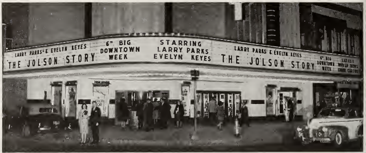
Spacious distribution of copy in two sizes of letters is shown in this display on the marquee of the Joy Theatre in New Orleans, La. The top fascia of the marquee consists in Wagner panels, and the letters are colored translucent plastic in 10- and 17-inch sizes.
