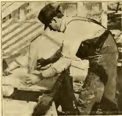
Laying Lapped Glass.
