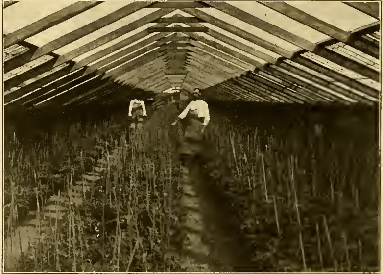
AT OTTO GRUNDMAN'S ESTABLISHMENT, SECAUCUS, N. J. Growing chrysanthemums in the open; showing enclosure with rafters and one row of sash covering.
