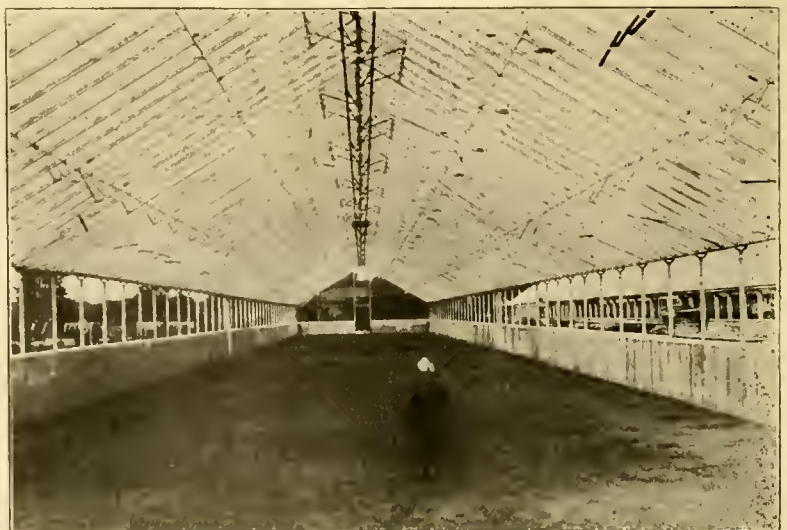
W. W. COLE'S NEW KING CONSTRUCTION HOUSE, AT KOKOMO, IND.
