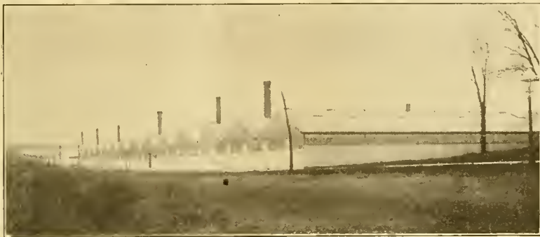
MAIN BLOCK OF GREENHOUSES AT PETER REINBERG'S, CHICAGO.
