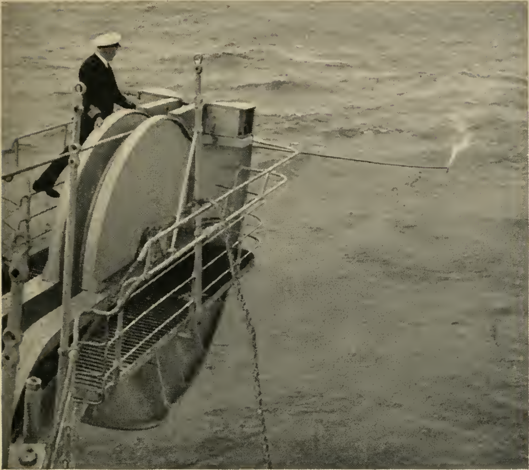
Fig. 9 — Cable payout over the stern.
