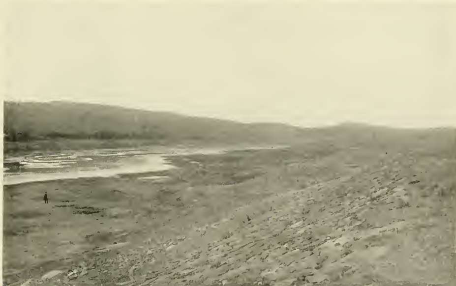
TUMBLEDOWN BROOK RESERVOIR (NO. 6) LOOKING NORTH.
