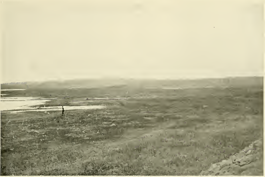
NO. 4 RESERVOIR LOOKING WEST.
