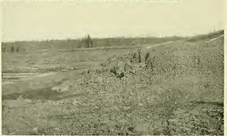
NO. 2 RESERVOIR, WEST AND EAST VIEWS.
