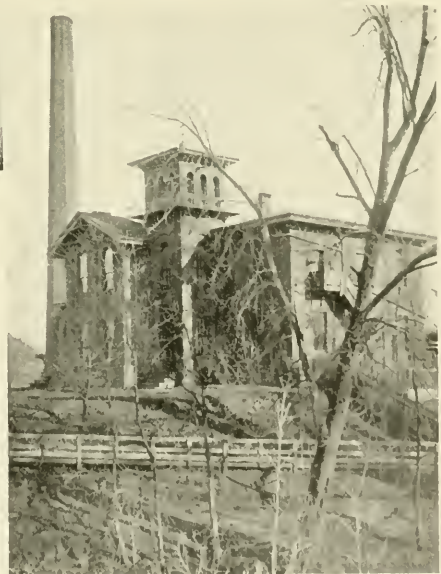
VIEWS OF THE GARDEN STREET RESERVOIR, THE CONNECTICUT RIVER WHERE WATER IS PUMPED INTO THE MAIN AND THE PUMPING STATION.
