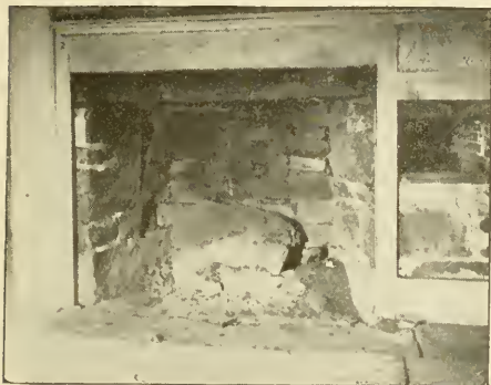
FIRE-PLACE IN HOUSE OF ALEXANDER JOHNSON.
