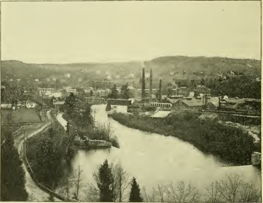
LOOKING SOUTHWEST FROM THE PARK.
