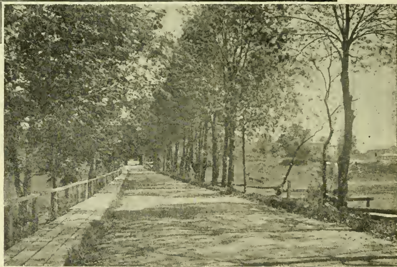
THE CAUSEWAY AND STONE BRIDGE.
