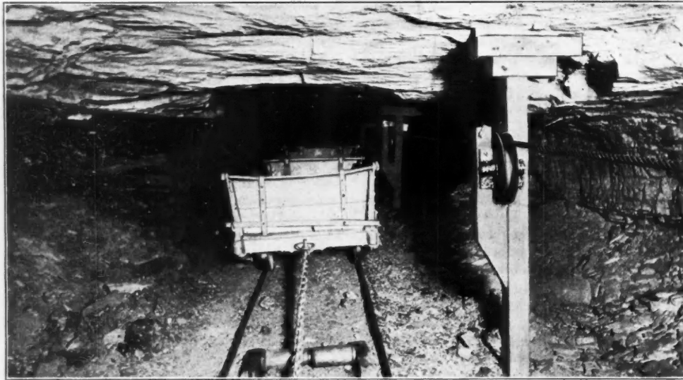
CHAIN CONNECTION, WOODEN ROLLER AND METHOD OF SUPPORTING TAIL-ROPE.
