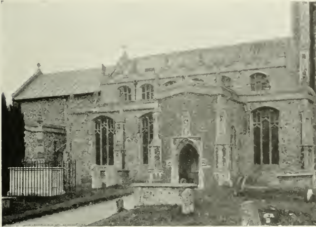
245. BRAMFORD, SUFFOLK. NORTH AISLE
