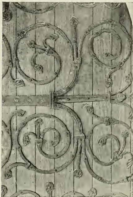
253. EATON BRAY, BEDFORDSHIRE
