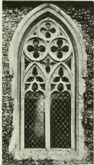
134 A SOUTH-AISLE WINDOW, RICKINGHALL INFERIOR, SUFFOLK
