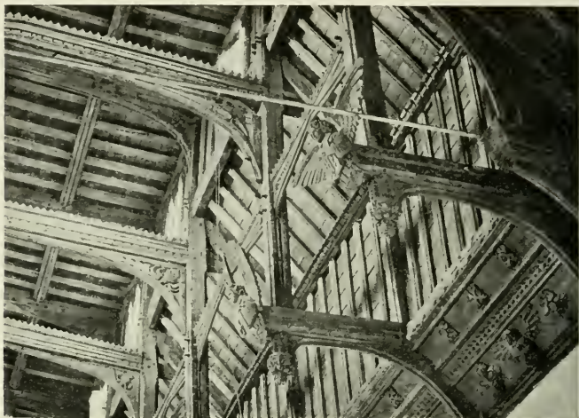
241. DETAIL OF ROOF, NEEDHAM MARKET
