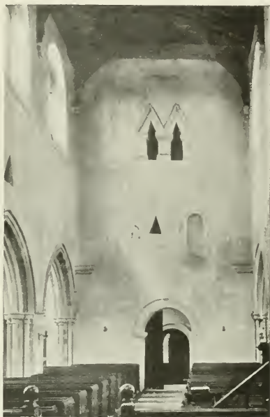
86. INTERIOR OF DEERHURST TOWER
