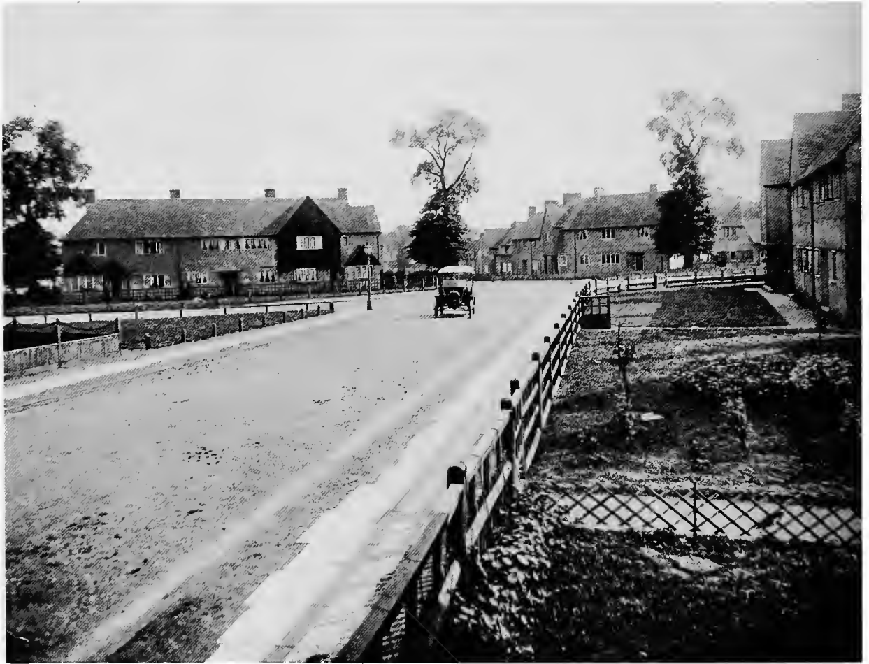
GOVERNMENT HOUSING SCHEME, WELL HALL, WOOLWICH. 1915. CONGREVE ROAD ( Boughton Road Crossing ) Looking South.
