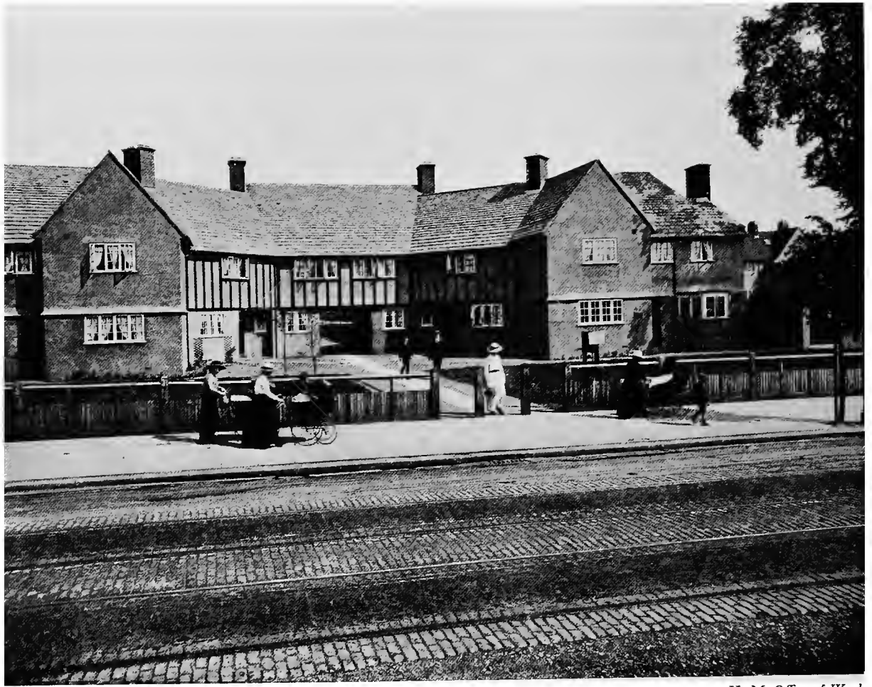
GOVERNMENT HOUSING SCHEME, WELL HALL, WOOLWICH. 1915. Entrance Group in WELL HALL ROAD, East Side.
