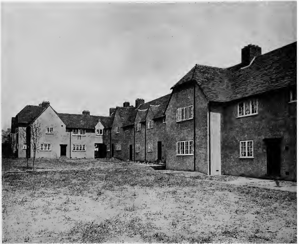
GOVERNMENT HOUSING SCHEME, WELL HALL, WOOLWICH. 1915. A Group in WHINYATES ROAD Looking North.
