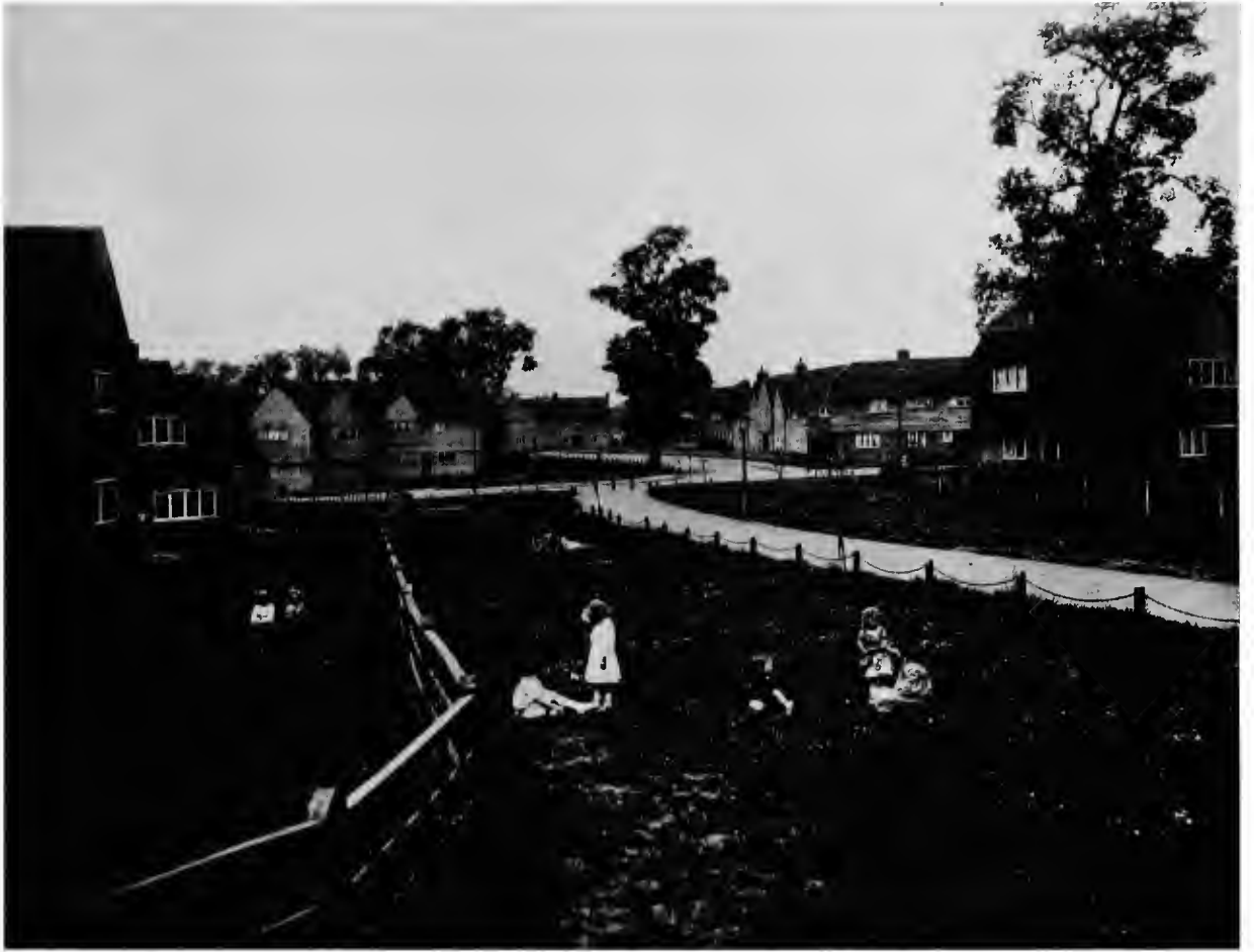
GOVERNMENT HOUSING SCHEME, WELL HALL, WOOLWICH. 1915. View of GILBORNE WAY Looking West.
