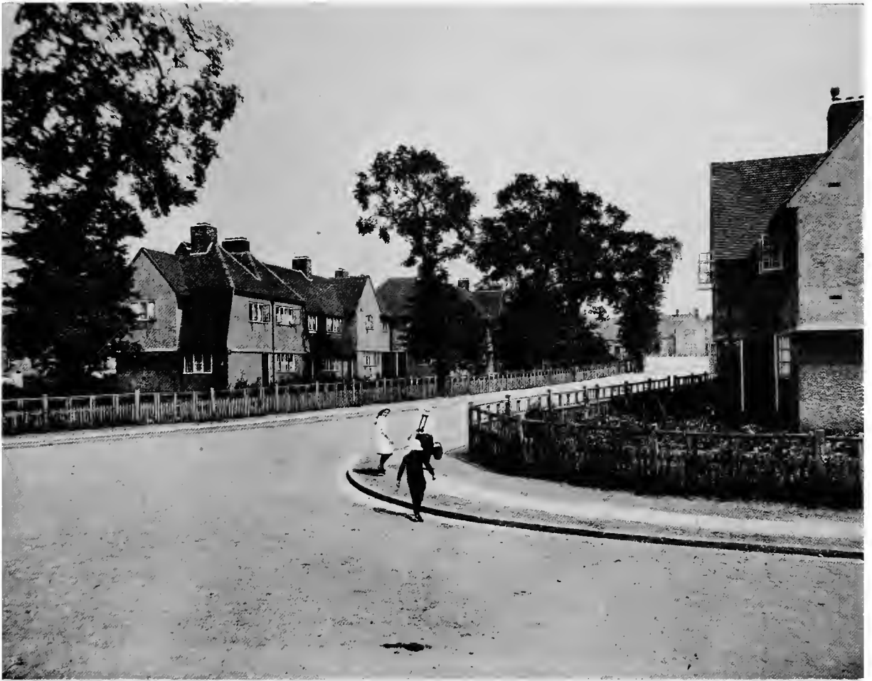
GOVERNMENT HOUSING SCHEME, WELL HALL, WOOLWICH. 1915. View in DICKSON ROAD Looking East.
