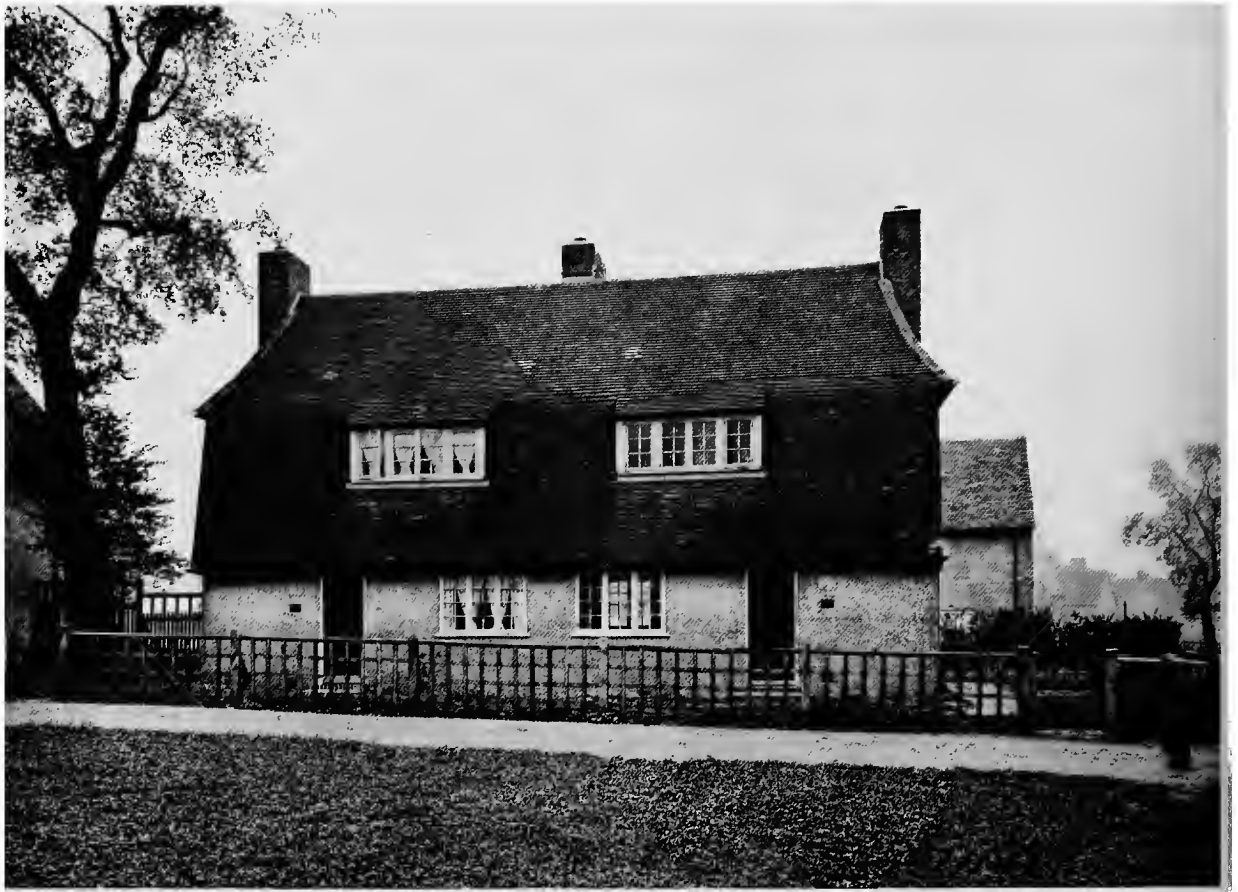
GOVERNMENT HOUSING SCHEME, WELL HALL, WOOLWICH. 1915. Pair of Cottages in LOVELACE GREEN.
