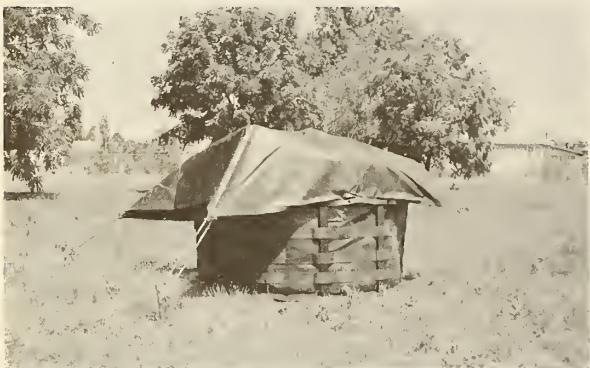
Four wooden tent pins are driven into ground to secure guy ropes attached to stave caps.
