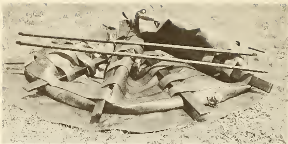
Tank with staves and caps attached and aluminum supports extended to diameter of tank.
