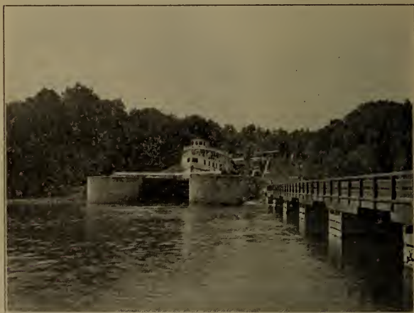
LOCKS AT JONES' FALLS, ON THE RIDEAU ROUTE—REACHED BY THE NEW YORK CENTRAL.
