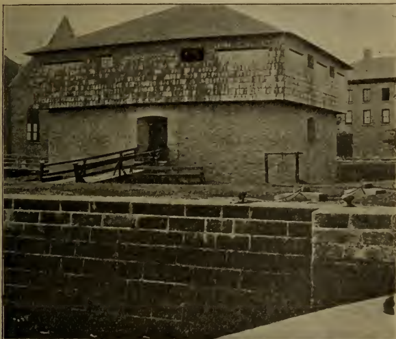
OLD MOATED BLOCK HOUSE, MERRICKVILLE LOCKS, RIDEAU ROUTE—REACHED BY THE NEW YORK CENTRAL.
