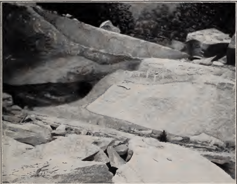
B. WEATHERING DUE TO GROUND WATER IN GRANITE QUARRY.
