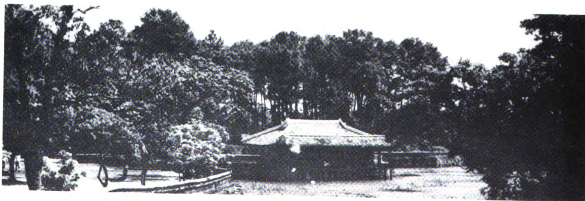
Entering the compound of the Emperor TU DUC tomb in Hue, Central Vietnam, one is captivated by the picturesque scenery of the pavillon built on piles where Emperor TU DUC (second son of THIEU TRI) used to come for relaxation.
