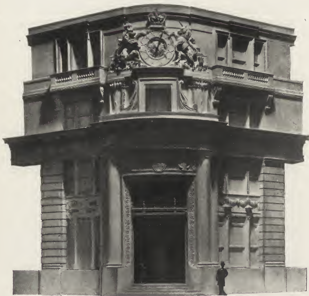
DETAIL OF THE ENTRANCE—ROYAL INSURANCE BUILDING.
