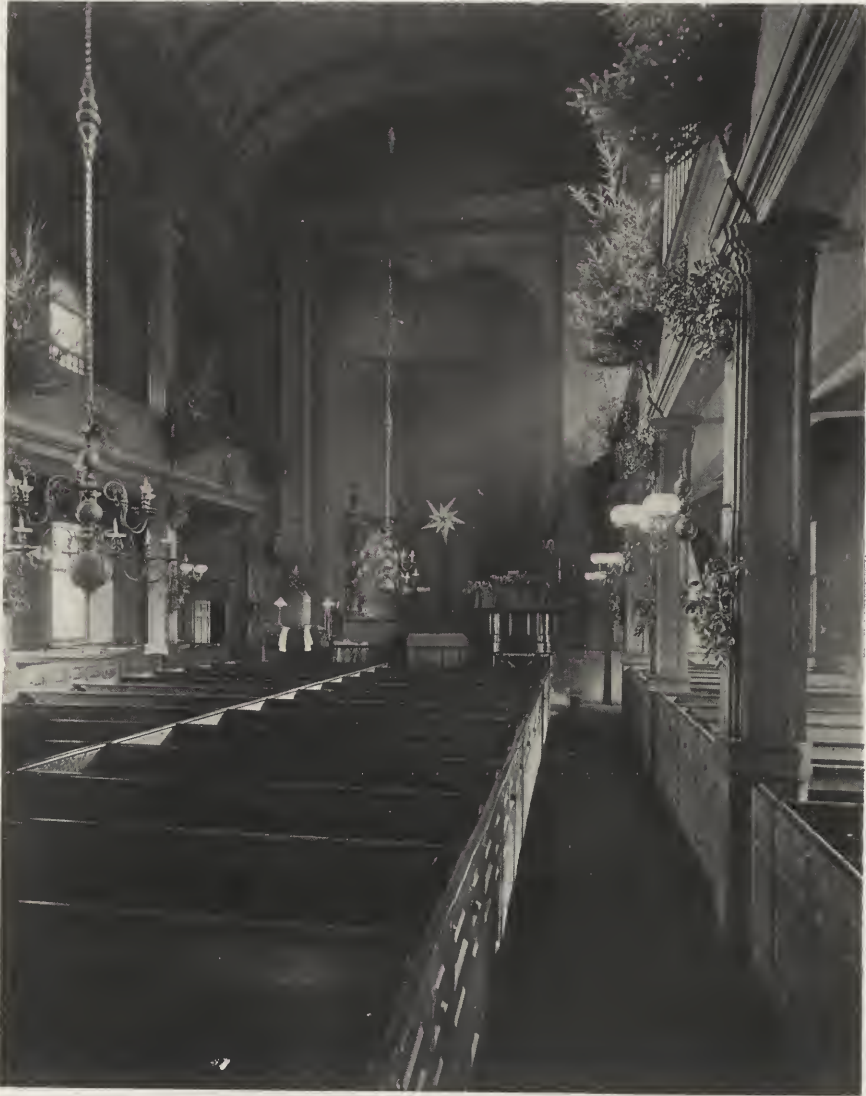
FIG. 2. GENERAL VIEW OF THE INTERIOR OF NORTH CHURCH. Boston, Mass.
