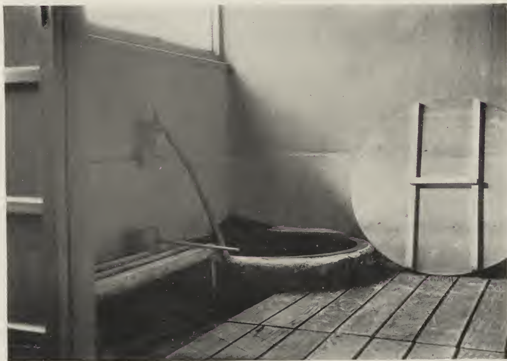
FIG. 23. BATHROOM IN PRIVATE HOUSE.
