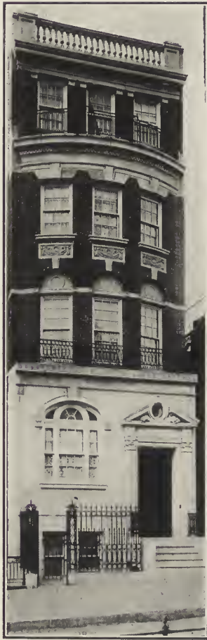
Fig. 14. "A Stilted Basement." No. 926 Park Avenue.
