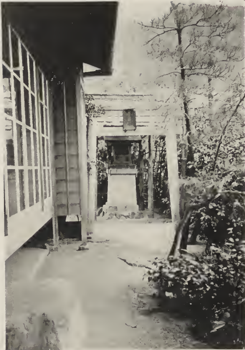
Fig. 3. The side of this house shows the way in which the posts rest upon exposed stones, which are slightly hollowed to receive them.
