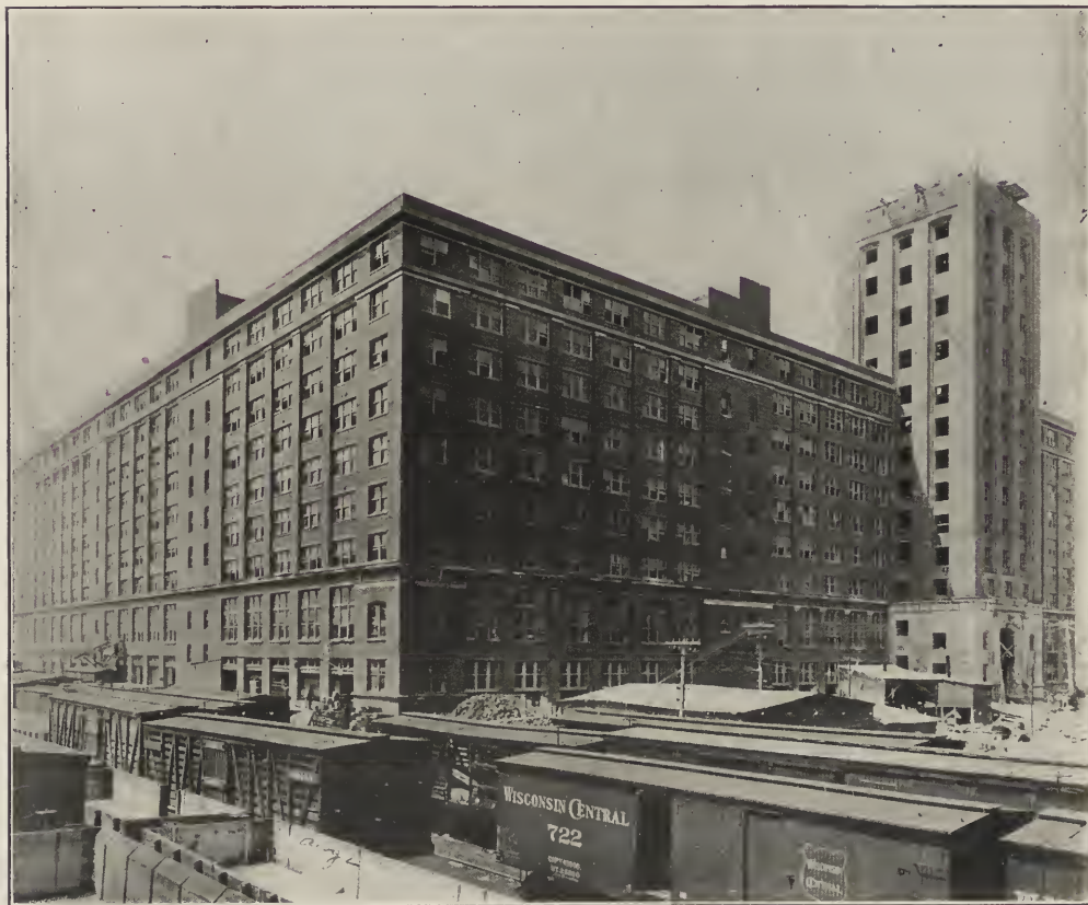
MERCHANDISE BUILDING, LOOKING NORTHWEST—SEARS, ROEBUCK & CO.
