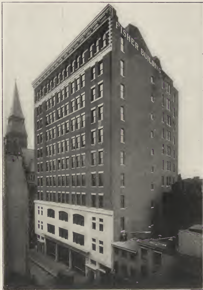
FISHER BUILDING, 97-103 EAST HOUSTON STREET, N. Y. CITY. Cream White Glazed Terra Cotta, Vellum Finish.
