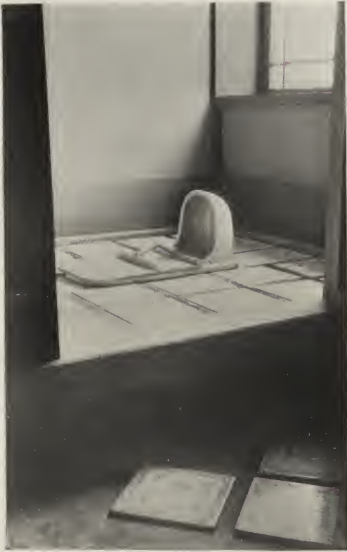
Fig. 18. Characteristic example of a private closet. The cement floor is paved with blue and white tiles. The opening is framed and protected in green porcelain. A natural twig has been used to make the handle of the cover.
