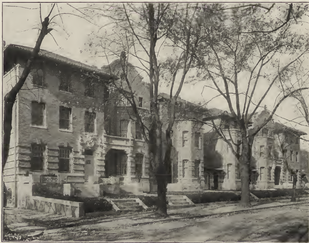
ROW OF RESIDENCES ON NINETEENTH STREET.
