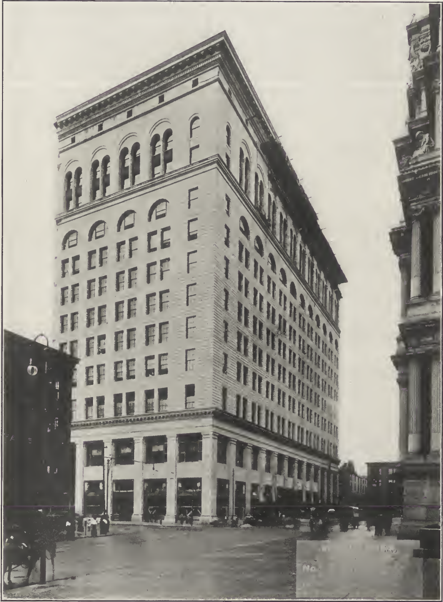
THE NEW WANAMAKER BUILDING.
