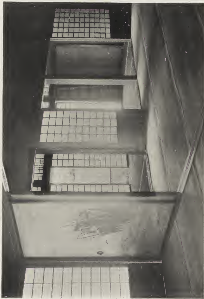
FIG. 13. A GOOD EXAMPLE OF THE ENCLOSED GALLERY CONTAINED IN THE BEST HOUSES. It is a protection against cold in winter, and enables visitors or servants to pass from one part of the house to the other with greater convenience.
