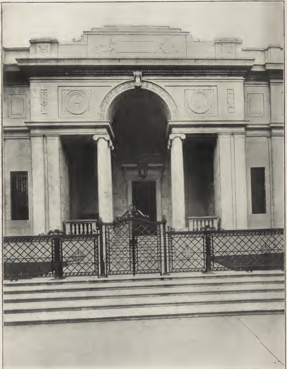
ENTRANCE LOGGIA—THE MORGAN LIBRARY AND ART MUSEUM. 36th Street, between Park and Madison Avenues, New York. McKim, Mead & White, Architects.
