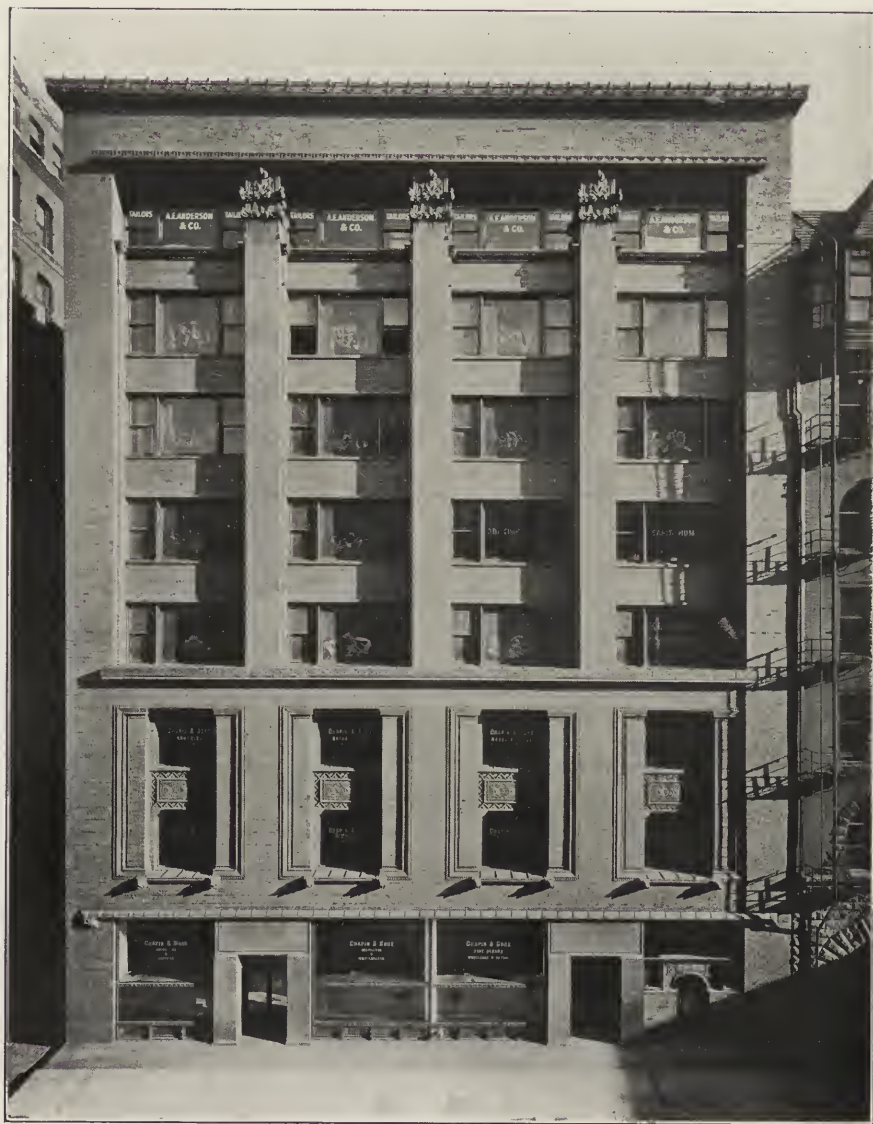
FIG. 3.—THE CHAPIN & GORE BUILDING.
