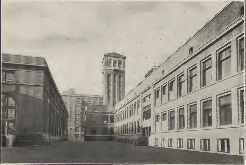
(1) ADMINISTRATION BUILDING. (2) COURT, WITH MACHINERY BUILDING ON LEFT. ADMINISTRATION BUILDING ON RIGHT—SEARS, ROEBUCK & CO.
