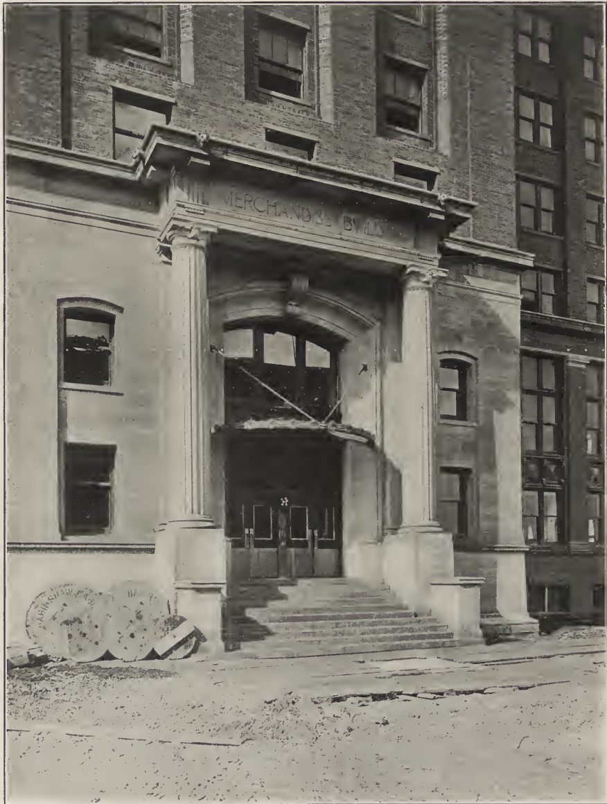
THE MAIN ENTRANCE TO THE MERCHANDISE BUILDING.
