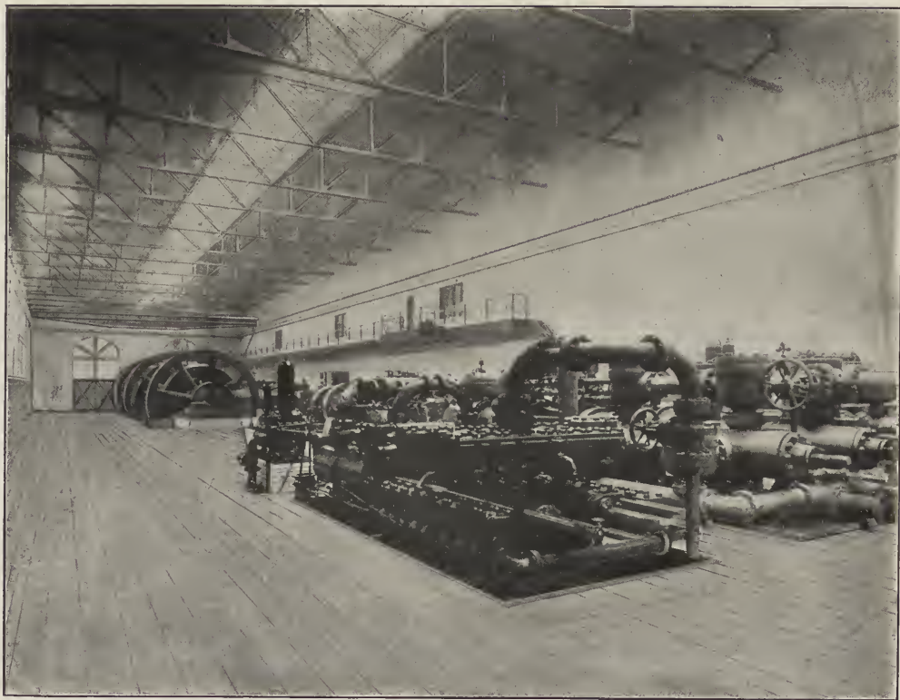
ENGINE AND PUMP ROOM—SEARS, ROEBUCK & CO. BUILDINGS.
