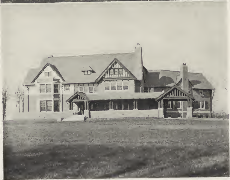
Figs. 13 and 14. The upper illustration is the house of Mr. E. C. Deardon, and the lower one is that of Mr. Geo. C. Blabon. Both houses are situated at Merion, Pa., and have been designed by Duhring, Okie & Ziegler.
