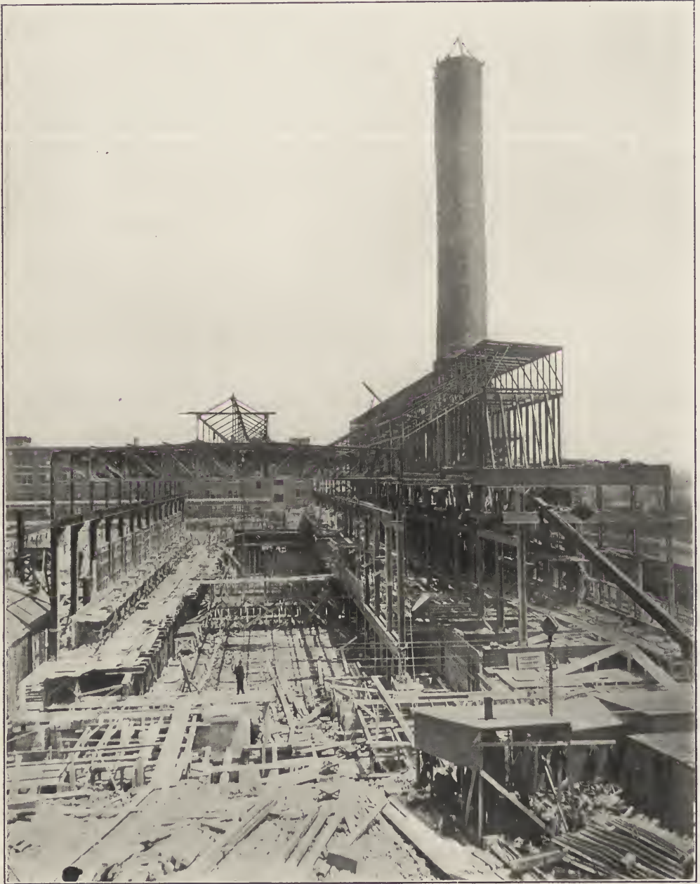
CONSTRUCTION OF THE POWER HOUSE—SEARS, ROEBUCK & CO.
