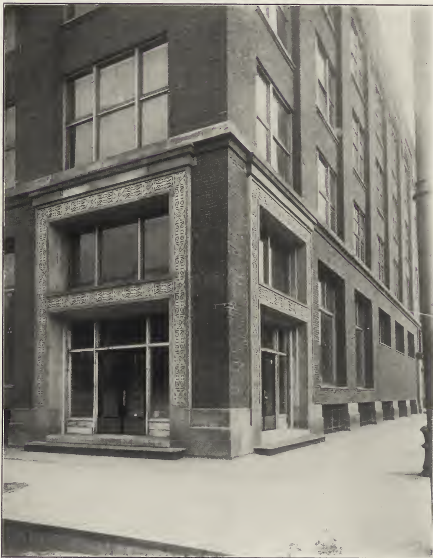
FIG. 4. THE DOUBLE CORNER ENTRANCE—BUILDING OF THE EASTMAN KODAK COMPANY Indiana Avenue and 18th Street, Chicago, Ill. Hill & Woltersdorf, Architects.
