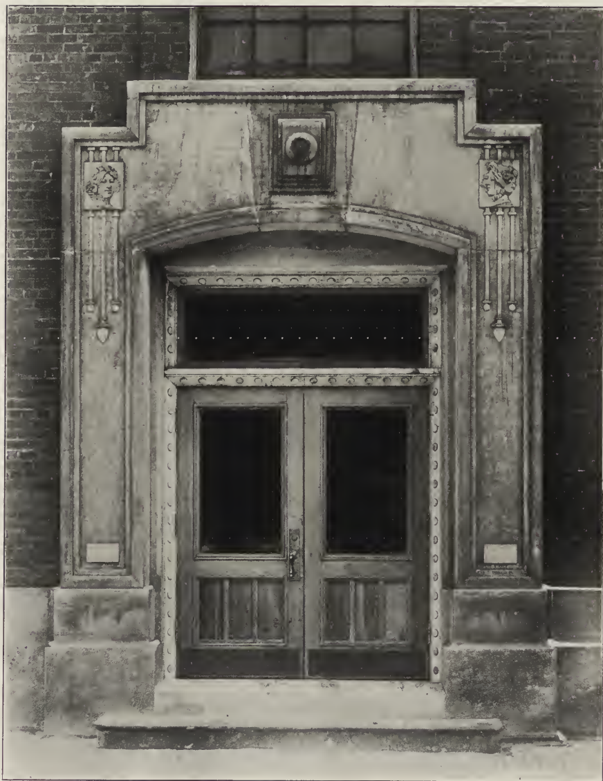
FIG. 5. THE INDIANA AVENUE ENTRANCE TO PASSENGER ELEVATORS AND PUBLIC STAIRS—BUILDING OF THE EASTMAN KODAK COMPANY.
