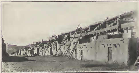
Fig. 2. Showing How the Successive Stories of the Houses Retreat, Acoma Pueblo, New Mexico.
