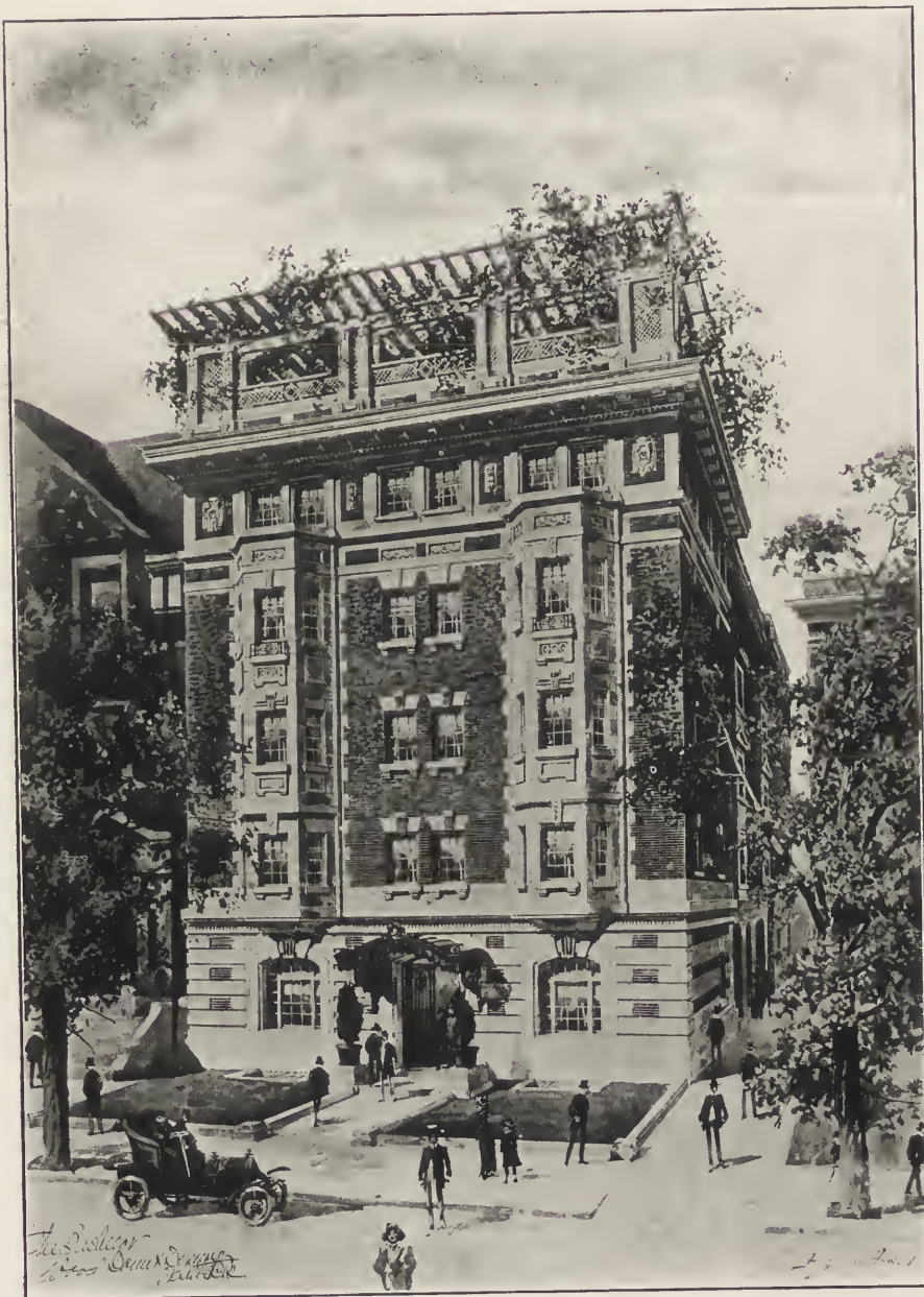
"THE BACHELOR" APARTMENT HOUSE.
