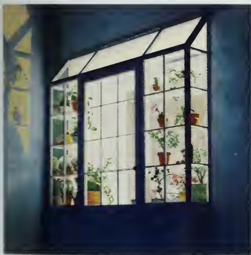
NIGHT-BLOOMING BEAUTY through Plate Glass adds to the appeal of this conservatory designed by Architect Earl W. Bolton, Jr. Windows with shelves of Plate Glass create an interesting effect. Picture windows, corner windows, glass screens and table tops are other ways to use the bright polished beauty of Plate Glass.
