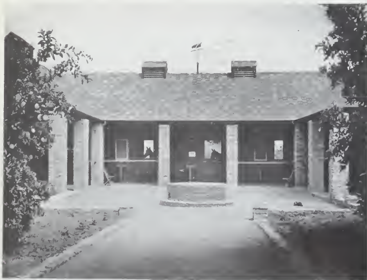
Close-up of center court of stables
