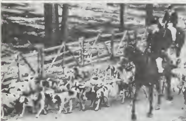
ENGLISH HURDLE FENCE made of hand split chestnut in sections 8'3" long, 4' high when erected. Twelve Hurdles make 100 feet of fence—640 Hurdles to the mile.
