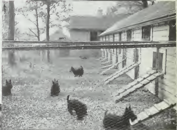
The kennels are air-conditioned and on either side of the indoor runway are individual kennels opening on the outside runs
