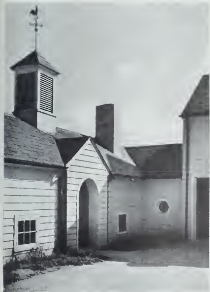
The upper stable court
