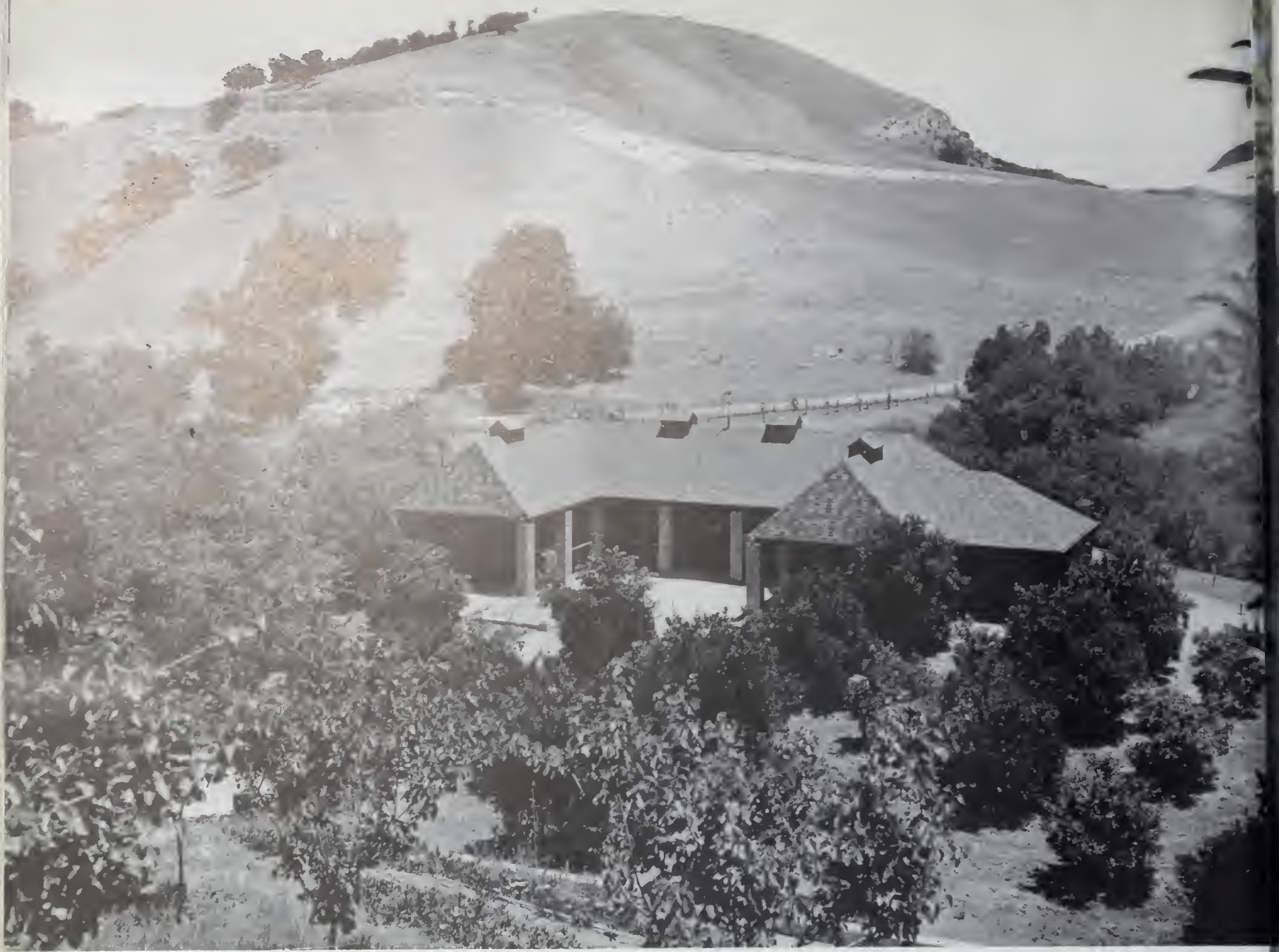
Looking down on the polo stables from the hillside above
