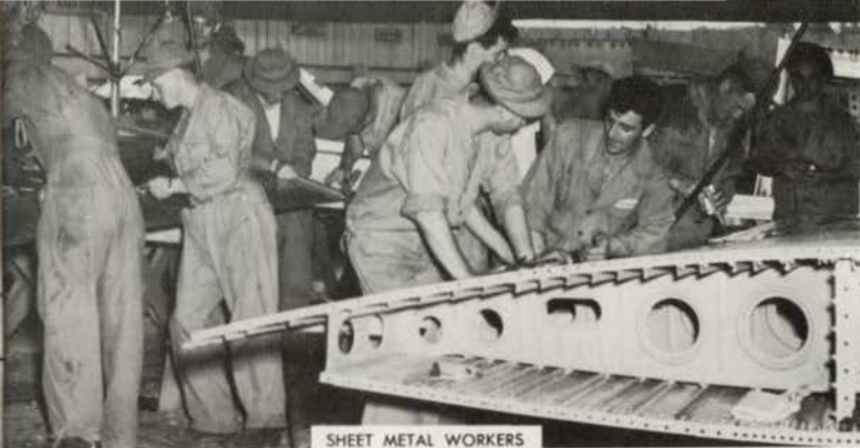
SHEET METAL WORKERS
