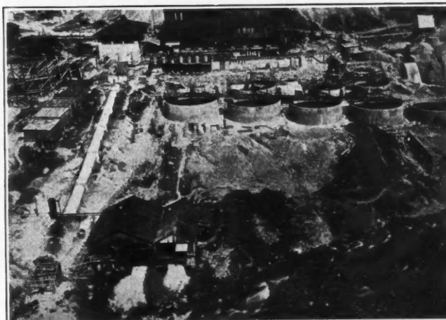
GENERAL VIEW OF PLANT BEFORE COMPLETION
