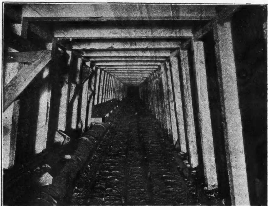
INTERIOR VIEW OF SPIRO TUNNEL, SHOWING CONSTRUCTION
