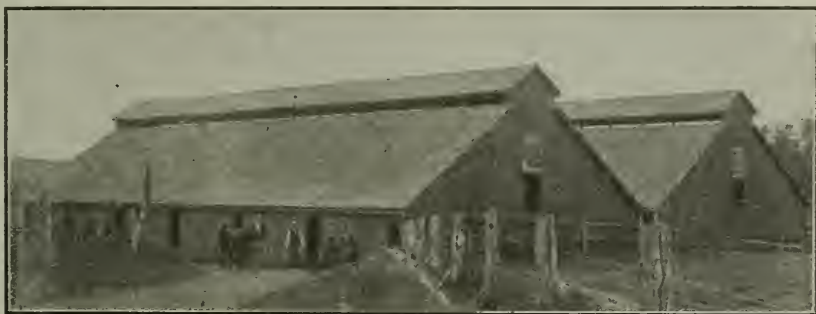
Co-operative Piggeries, showing ventilators open at the top and ends, and the driveway at the end of the gutter, where the litter is carried away in a tank wagon.
