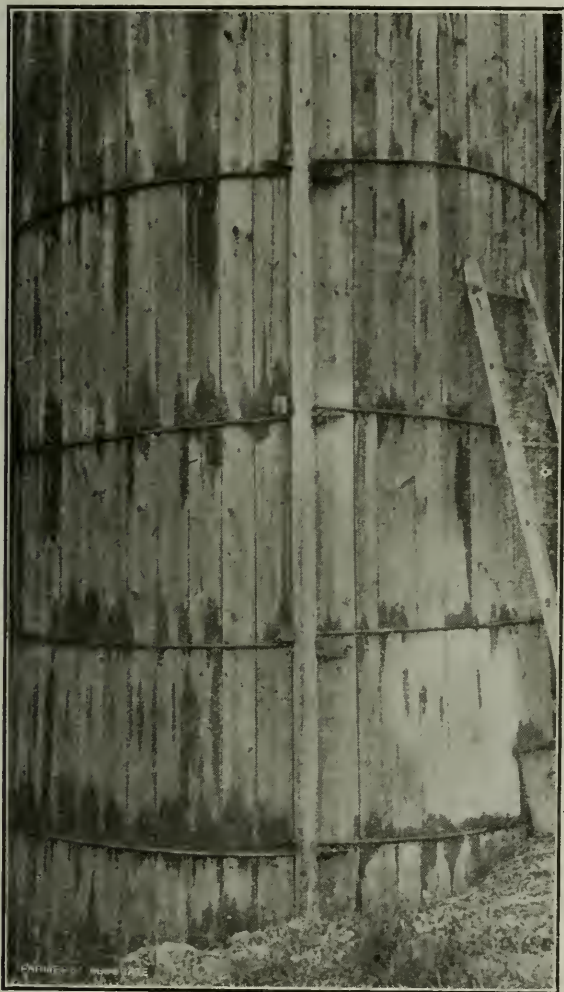
Common Stave or Tub Silo. Note the 4-inch by 4-inch studding used for holding the hoops in place. The durability of this silo could be increased by raising the staves off the ground.
