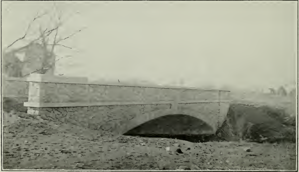
Usher Creek Bridge.
