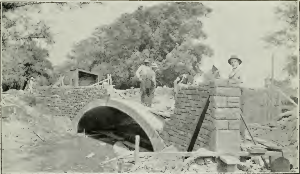
Baker's Creek Bridge. (Under construction.)
