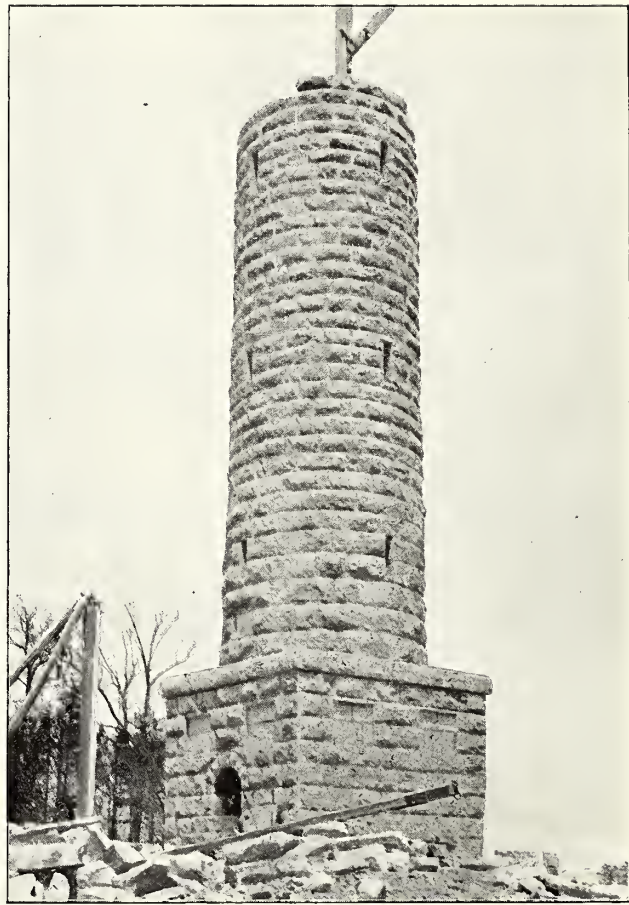
General Wilder's Monument During Construction.
