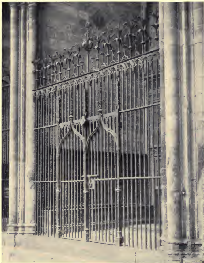
FIG. 16. REJA OF A CLOISTER CHAPEL. Barcelona Cathedral.
