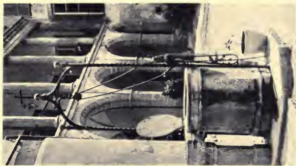
FIG. 148. ARMADURA OR WELL CRANE. Palma. XVII Century.
