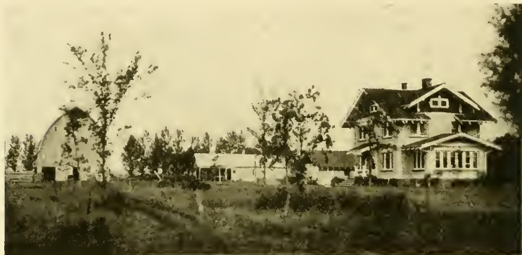
FIG. 81. VIEW FROM MAIN ENTRANCE
