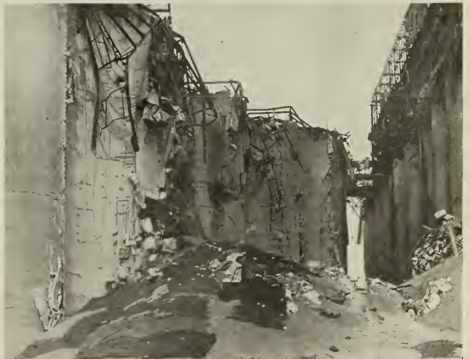
THE DEMOLISHED TANKS AT SOUTHEAST CORNER OF THE STORAGE HOUSE
