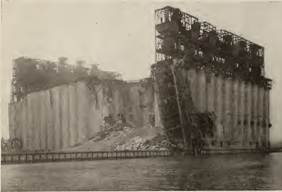
THE ELEVATOR AFTER THE EXPLOSION General View of the Plant from Across the Calumet River, looking Northwest
