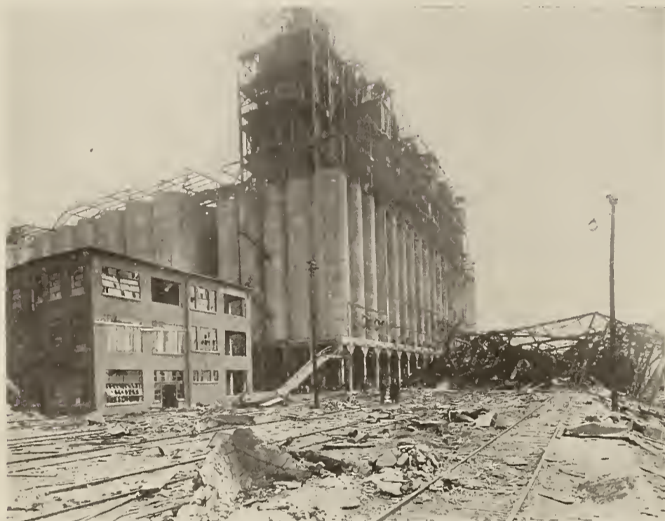
ANOTHER VIEW OF THE ELEVATOR AFTER THE EXPLOSION View Looking Southeast; Office to the Left, Track Shed Debris to the Right
