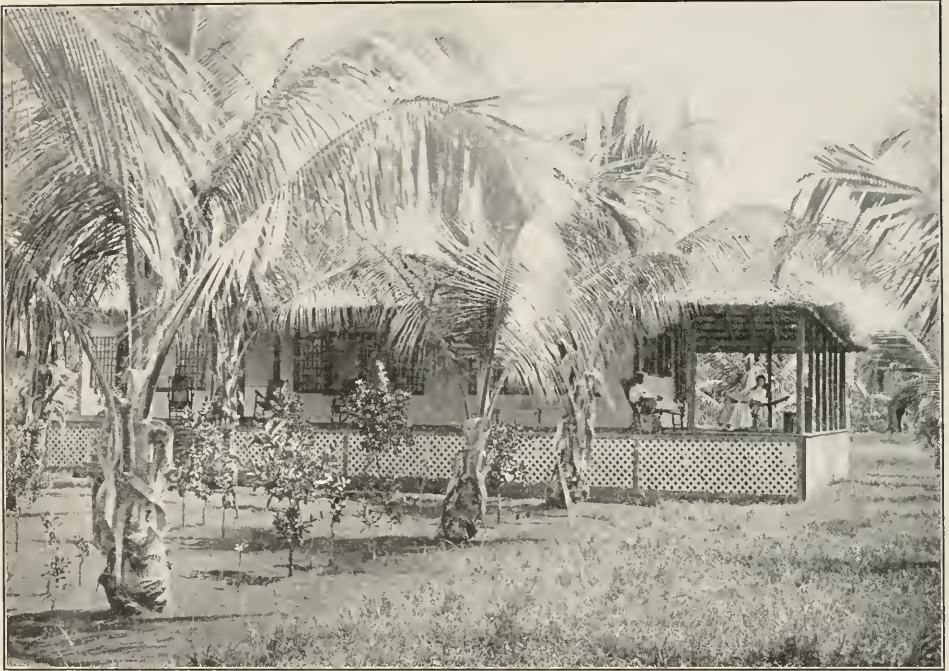
AMERICAN HOMES IN CUBA. Residence of Chas. E. Hall in La Glorta. Built of native woods; palm thatched; twelve-foot porch on three sides; six rooms, kitchen and bathroom. Approximate cost between $2,500 and $3,000.
