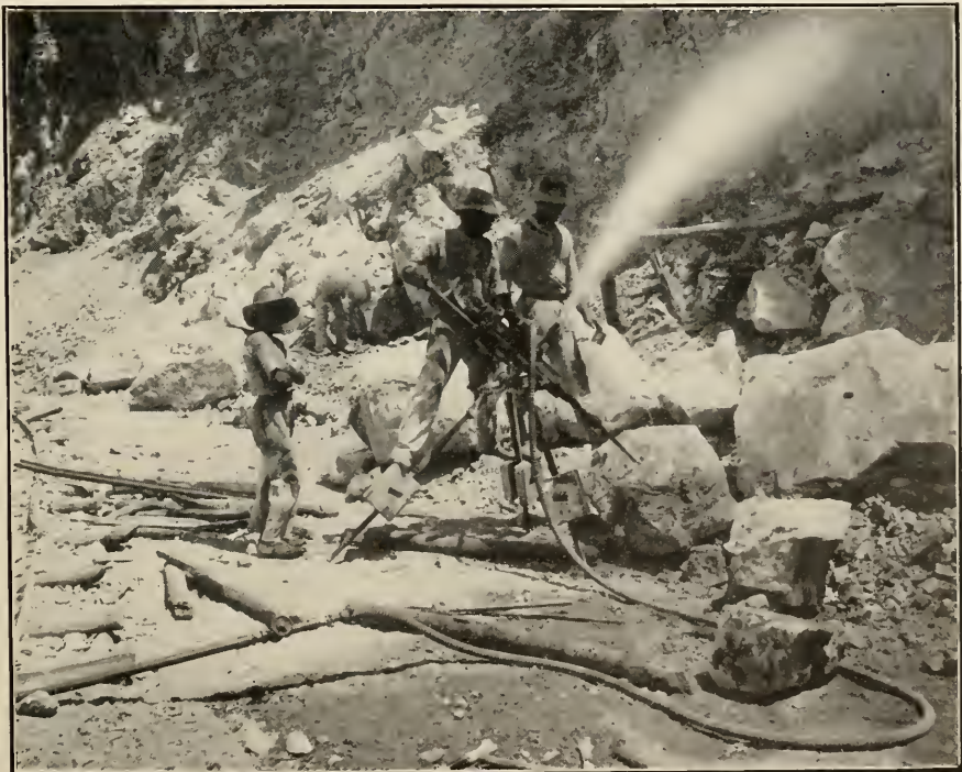
Steam drill at work at the Daiquiri Mines, Oriente Province.
