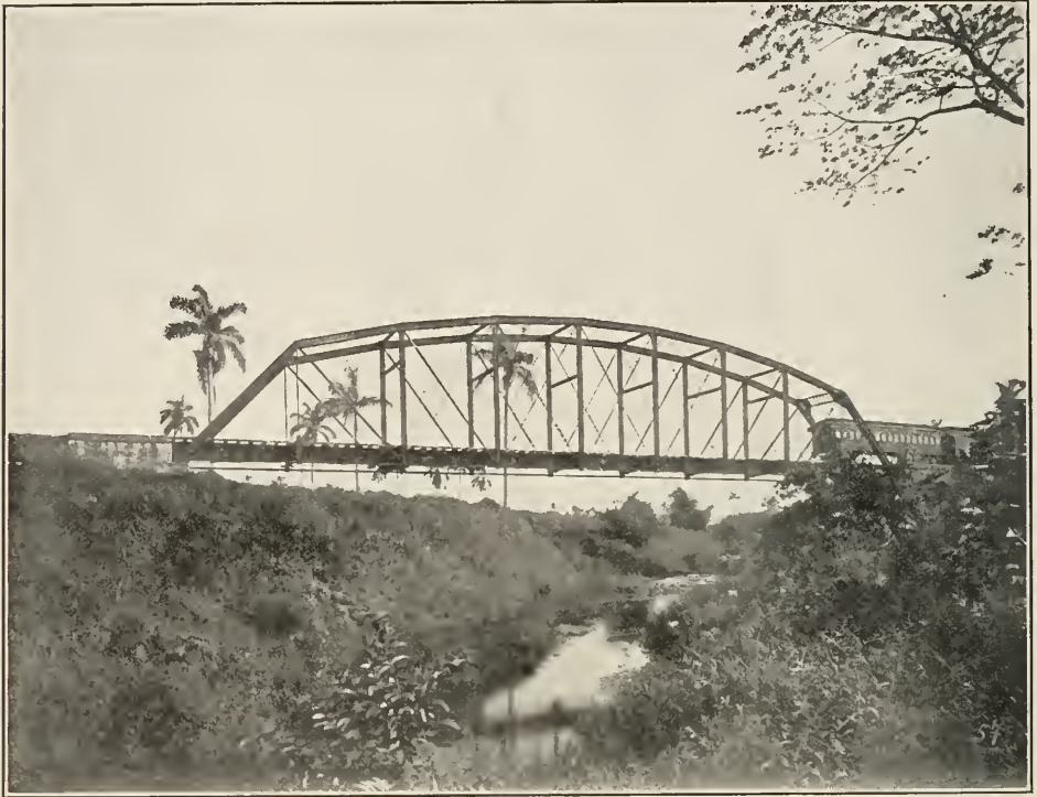
Bridge over the Sagua River, Sagua la Grande.
