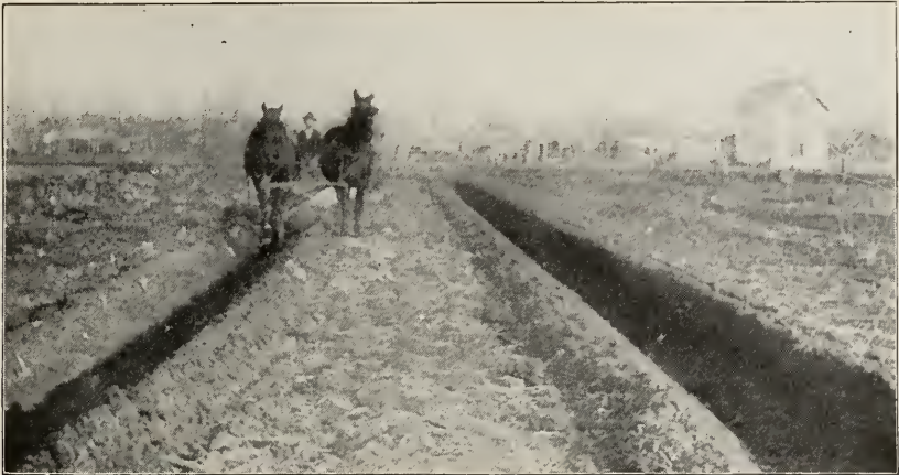
Making two "V"-shaped ditches, each 30 inches wide and twenty inches deep. The adjustable seat allows an upright position while the machine is on an angle.
