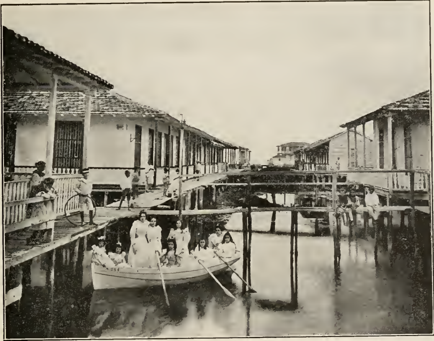
Scene at Isabella de Sagua, the port of Sagua la Grande on the north coast, and one of the streets. Important improvements are under construction here.
