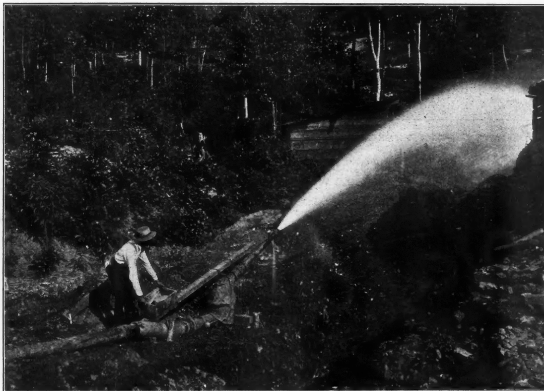
HYDRAULICKING AT CROWN MOUNTAIN MINE, NEAR DAHLONEGA, GEORGIA.
