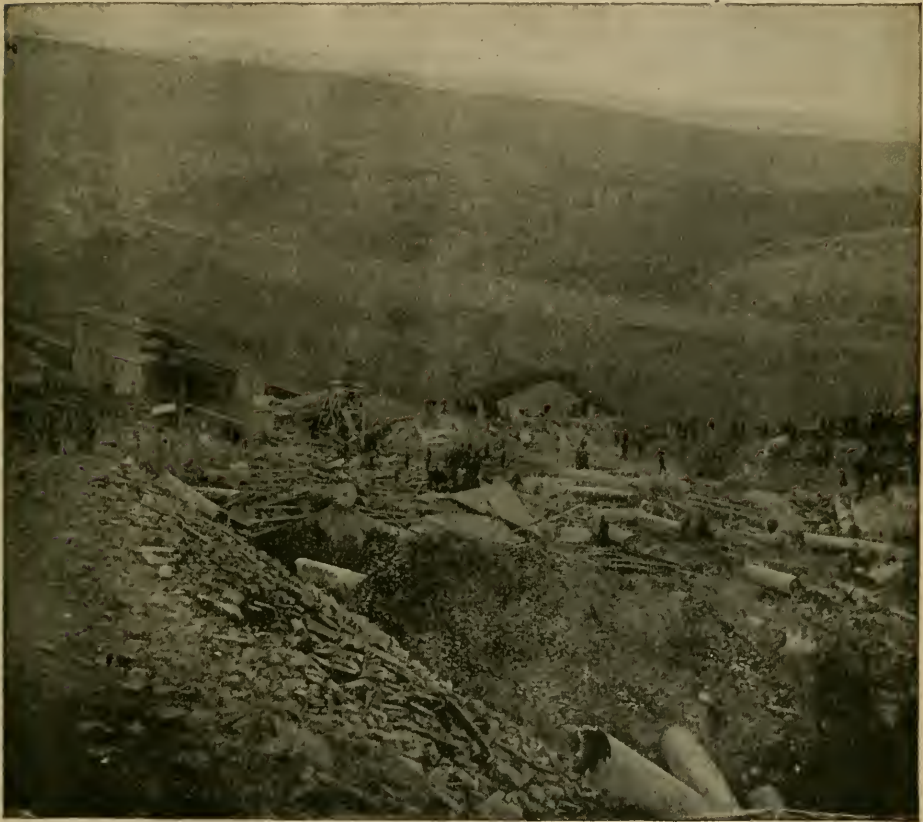
GENERAL VIEW OF THE RUINS.
