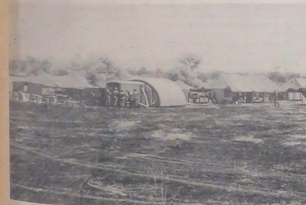
DECONTAMINATION ZONE —Behind the small inflatable "tent" and the tent to its left, is the "decontamination line." All casualties supposedly contaminated by nuclear, biological or chemical agents are brought here first for treatment and decontamination before they are allowed into the rest of the hospital area. The inflatable buildings are supposed to be able to resist fallout from NBC warfare.
