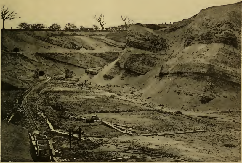
FIG. I.— VIEW OF STOCKINGFORD CLAY-PIT, SHOWING THE THICK COAL.
