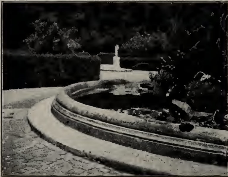
Water basin at the Villa Medici, Rome.
