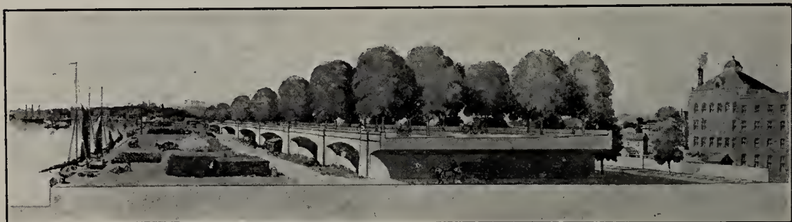
No. 10.—Typical treatment of Potomac Quay.
