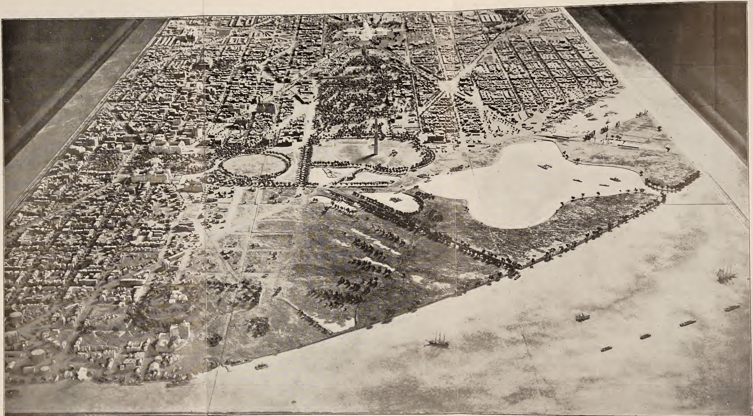
NO. 34.—MODEL OF THE MALL, SHOWING PRESENT CONDITIONS. LOOKING EAST.
