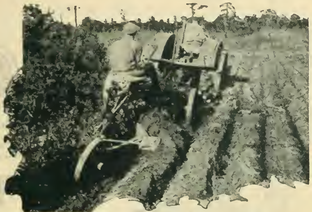
Flowing New Ground Turf After Stumps Have Been Removed.
