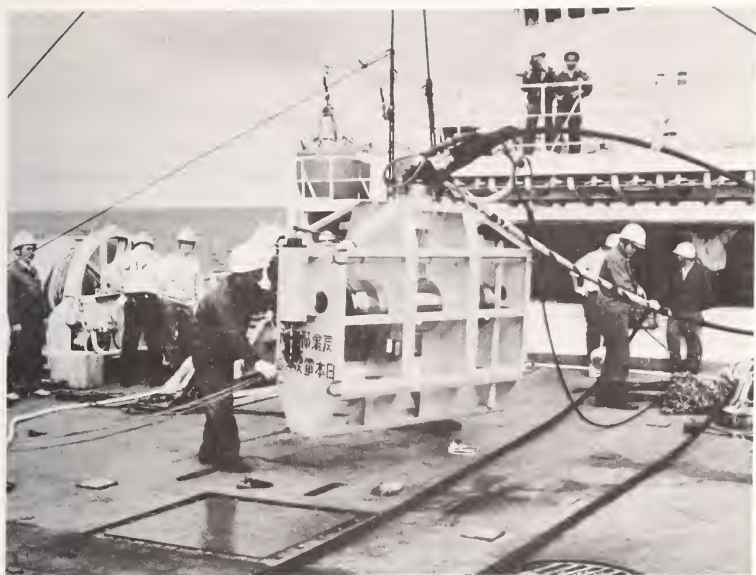
Figure 10 Trial Layings of the Terminal Apparatus
