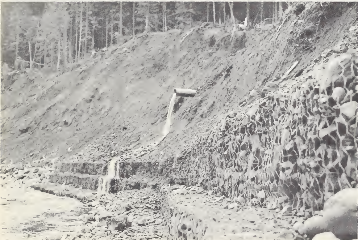
Photo 26.--A creek bank and rural road protected by wire-bound rock riprap, subbasin 9. Survey Party photo. 7-1378-8
