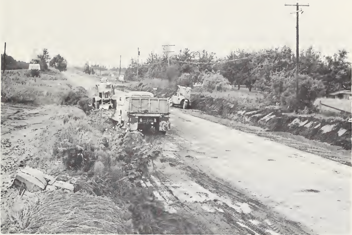
Photo 31.--A Multnomah County road crew is removing sediment from N. E. Halsey St., subbasin 11. SCS photo. F-128-8
