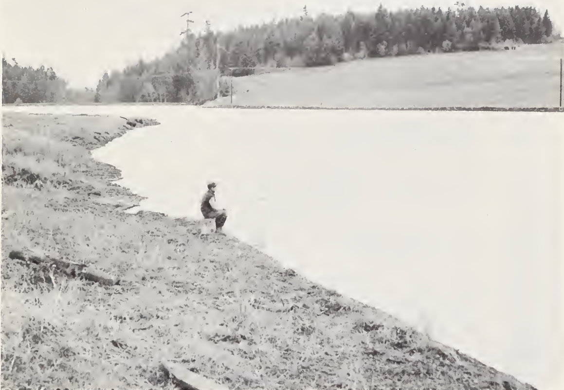
Photo 36.--A typical medium sized reservoir constructed for multiple use in subbasin 8. SCS photo. 7-616-12
