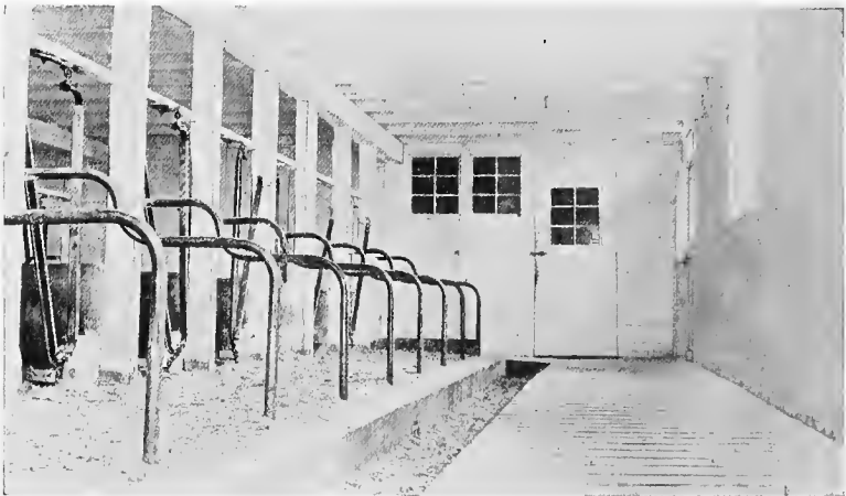
Fig. 97.—Side aisle of certified milk dairy transformed from old barn at small expense.
