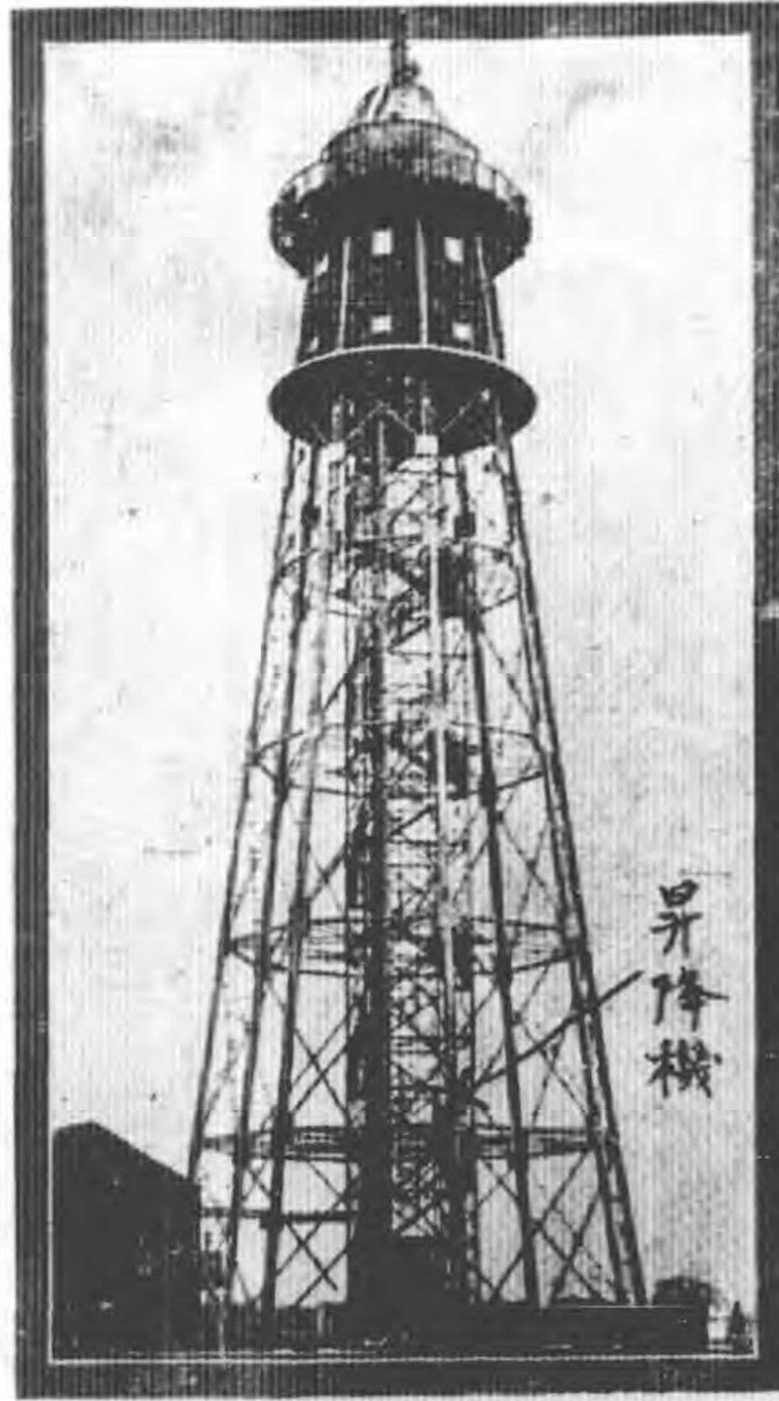
New mooring mast at Cardington, England, build for the giant dirigible, R101.
