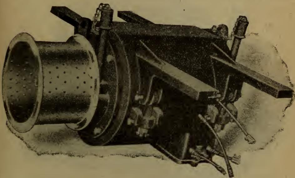
FIG. 73. GENERATOR SHOWING PERFORATED PULLEY AND SUPPORTING ARMS.
