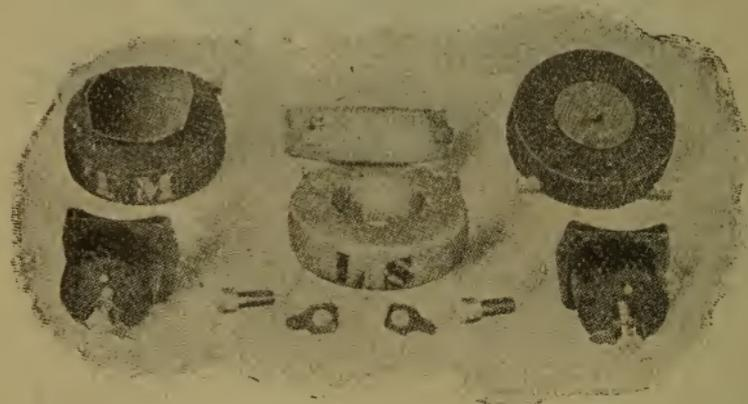
FIG. 89. BUCKER FIELD COILS AND POLE PIECES.
