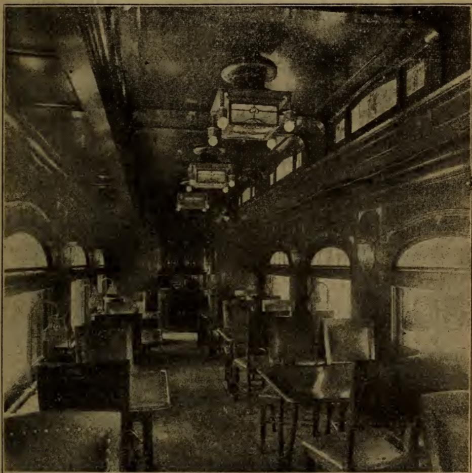
FIG. 58. INVERTED BURNER LAMPS IN DINING CAR.
