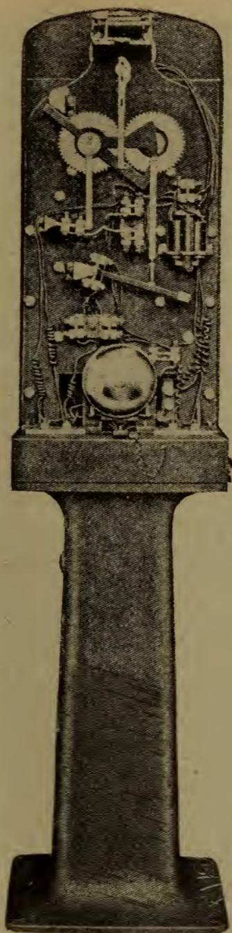
FIG. 123. ABSOLUTE STAFF INSTRUMENT WITH PEDESTAL.
