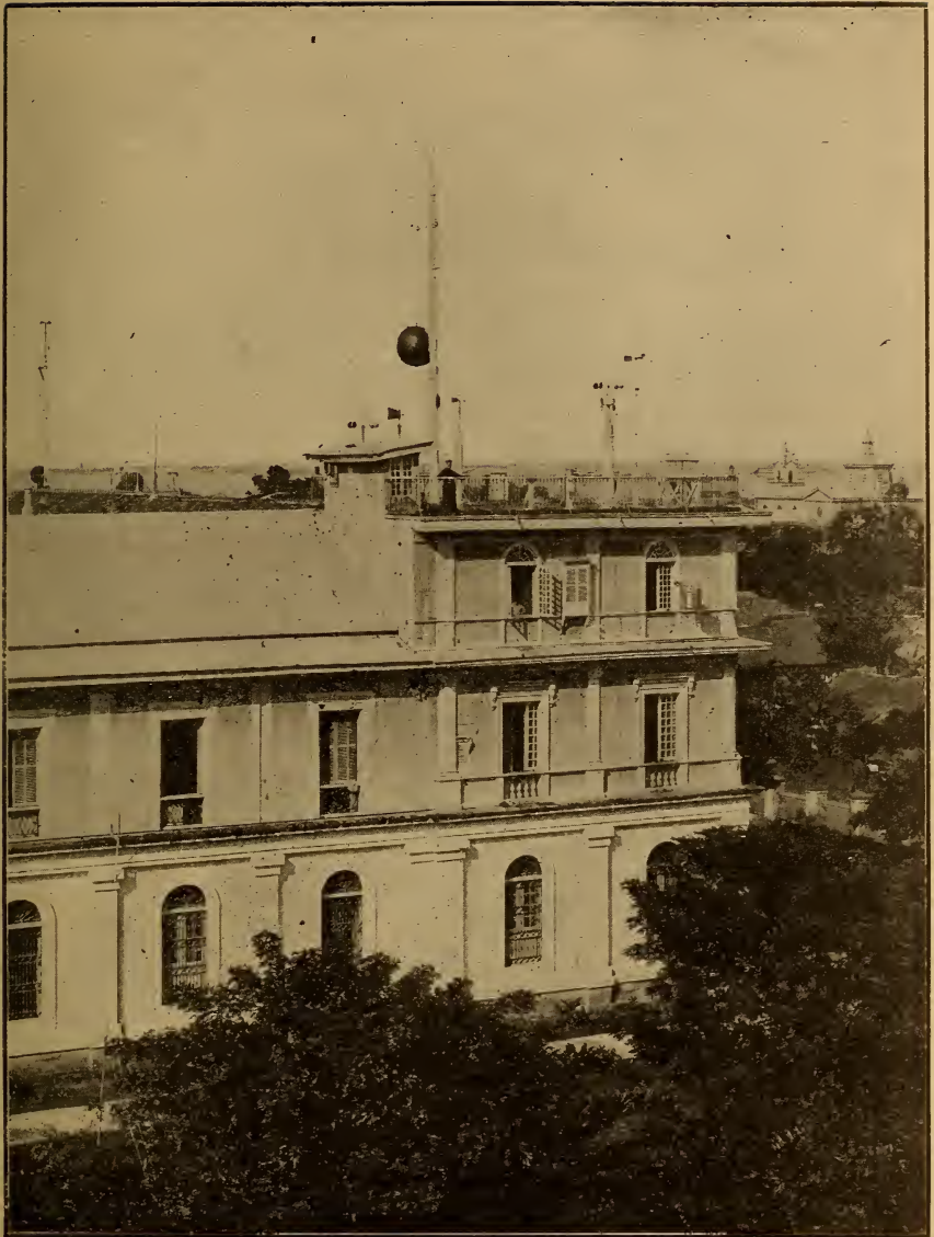
DEPARTMENT OF SEISMOLOGY AND TOWER OF METEOROLOGICAL APPARATUS. Manila Observatory.
