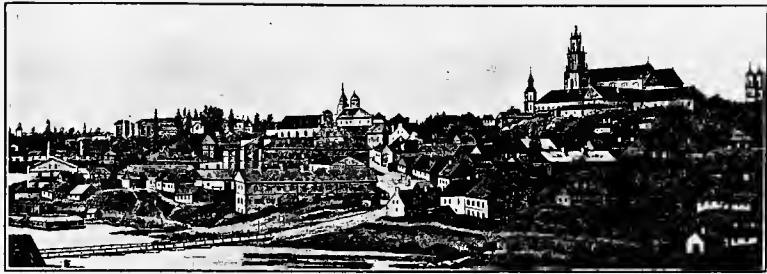
FIG. 32.—GENERAL VIEW OF GRODNO
