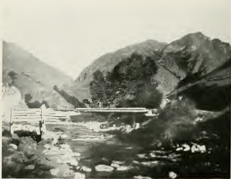
CANTILEVER BRIDGE ON THE ROAD TO LABRANG
