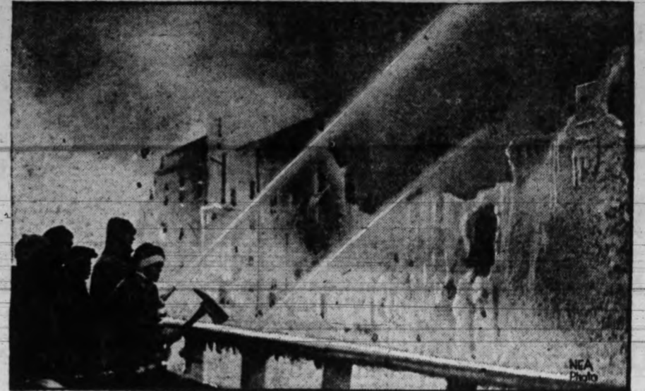
Freezing point temperature, causing streams of water to congeal in icy mass on the walls of the burning structure seriously hampered the work of firemen when they battled the recent blaze which destroyed Omaha, Neb., packing plant of Armour & Company. Loss is believed to have been well over a million.
