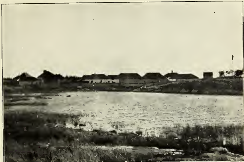
FIG. 1.—GENERAL VIEW OF NORWAY HOUSE.
